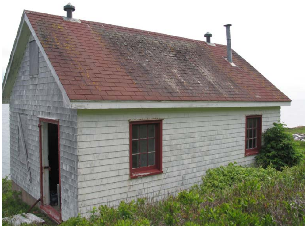
Figure 2. North and East walls of CWS cabin. (A. Campbell photo)
