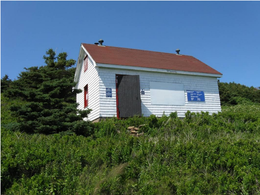
Figure 4. South wall of CWS cabin with new NWA Boundary, Public Notice and 2' X 4' signage installed. (A. Kennedy photo)
