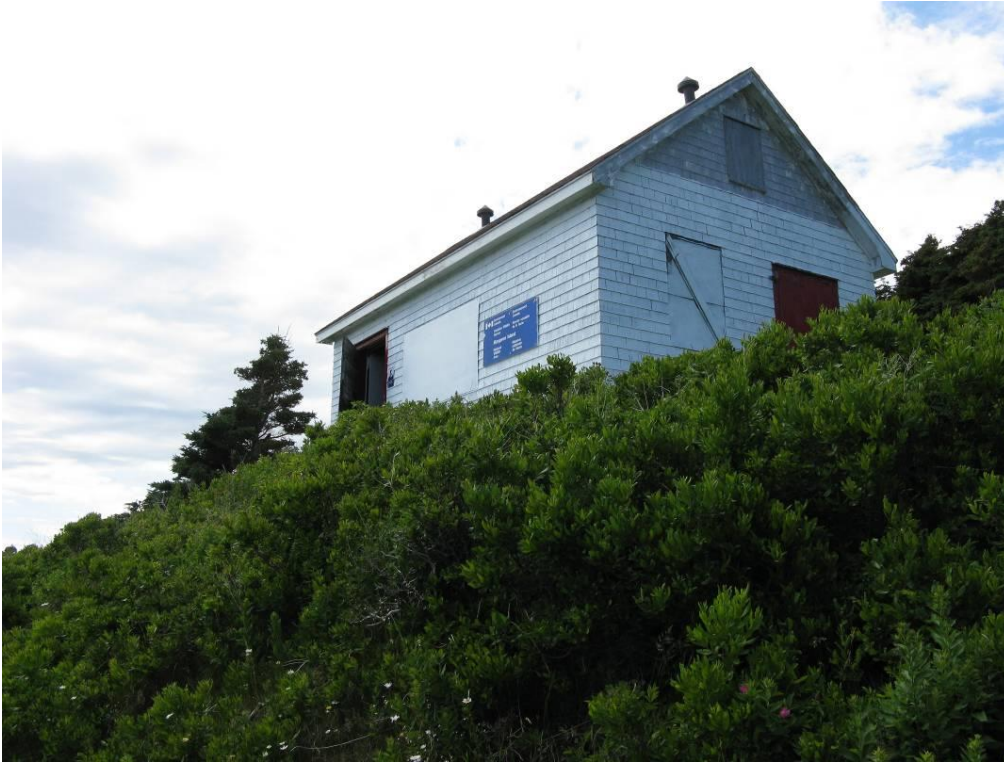
Figure 3. East wall of CWS cabin, rear door boarded up. (A.Kennedy photo)
