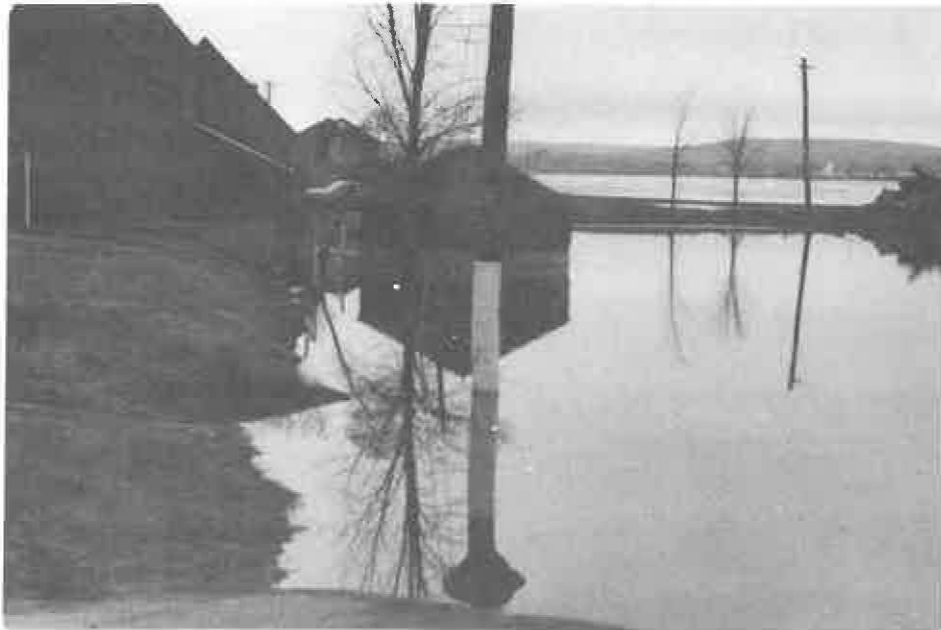
Fredericton Pumping Station, approximately at peak, Monday, April 30, 1979, at 5:00 p.m.
