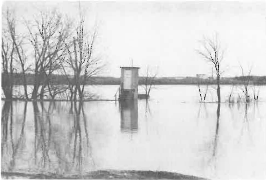
Maugerville Gauging Station, just before Burton Bridge, May 1, 1979, at 8:42 a.m.
