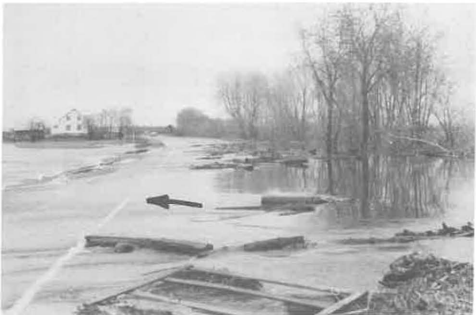
Debris on T.C.H., looking downstream about 1.0 mile below Burton Bridge, April 30, 1979, at 11:30 a.m.
