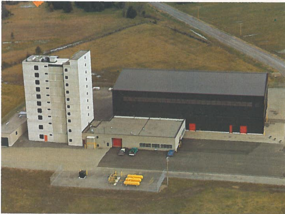
The Fire Research Field Station, located near Carleton Place, Ontario.
