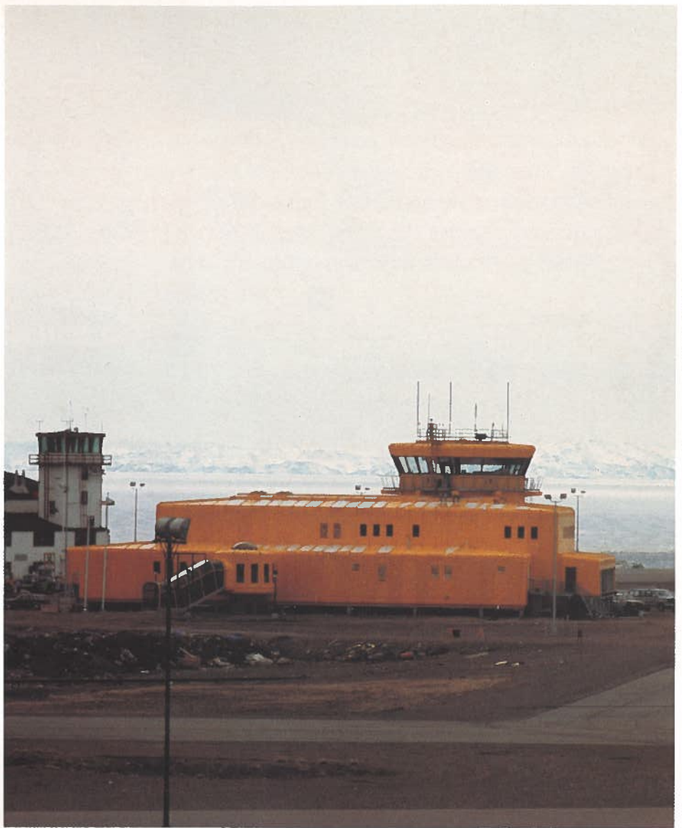
Plastics-clad airport terminal in Frobisher Bay, Northwest Territories.
