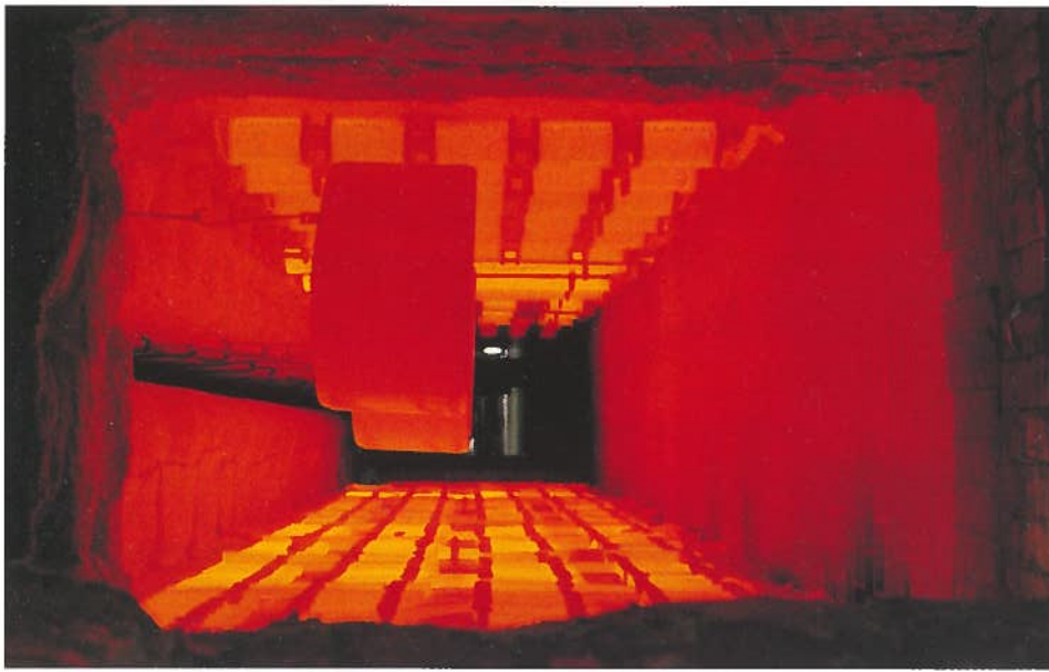
Washer parts traveling through an electrically heated porcelain enamelling furnace.
