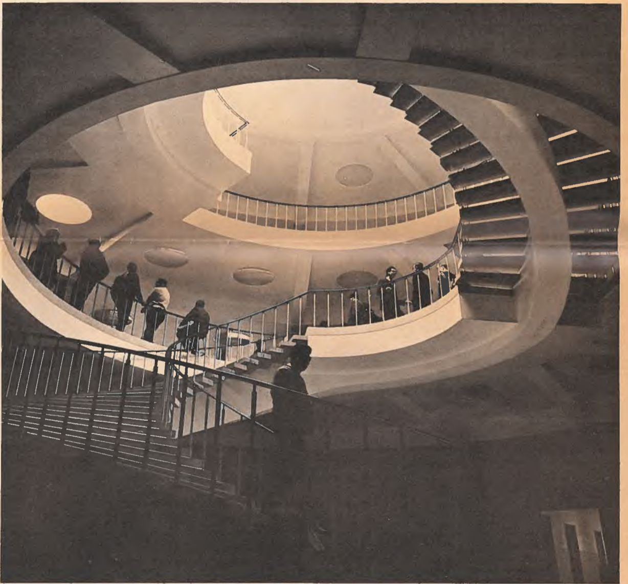
Many construction chemicals were used to build this staircase; chemical specialties are essential to the construction industry.
