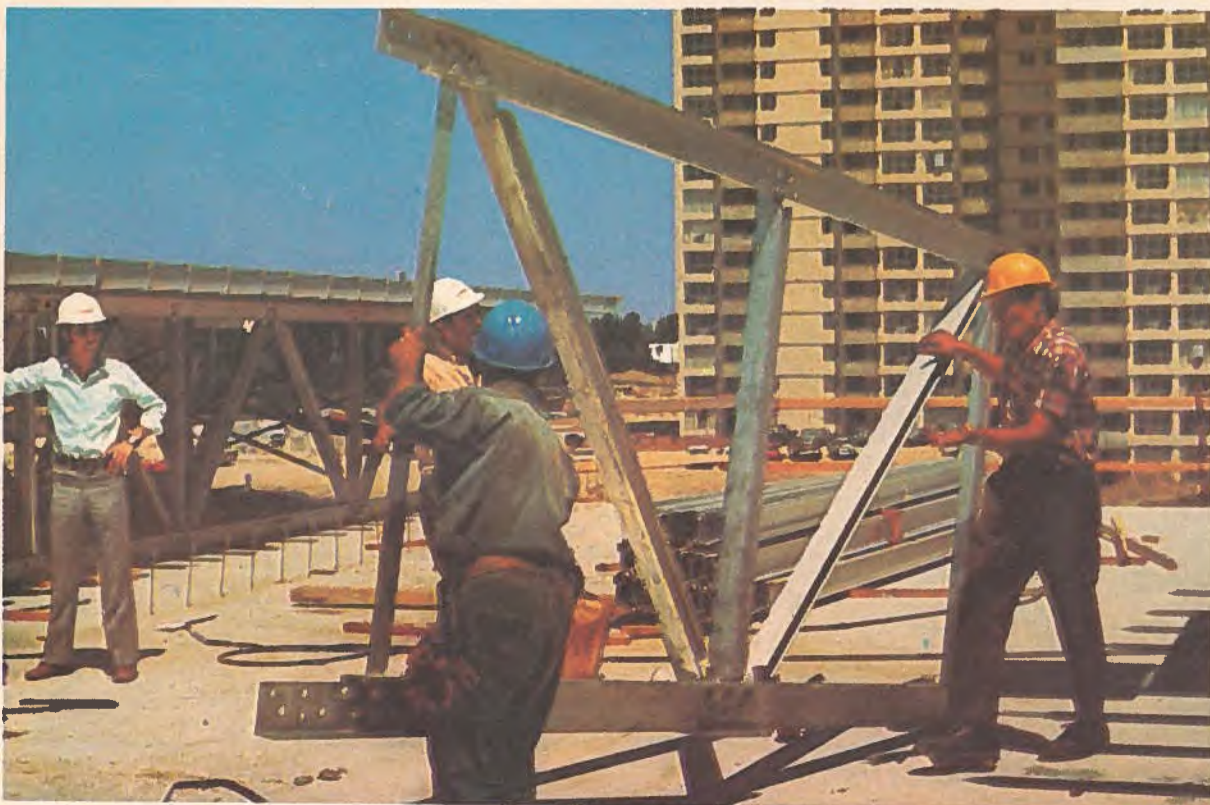
Aluma Building Systems on the job at a high-rise building site.
