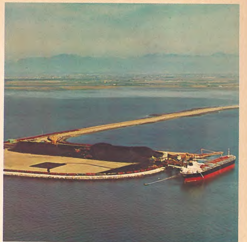
The Roberts Bank Superport off Canada's west coast. This huge facility handles rail car unloading, stockpiling, reclaiming and shiploading. Swan Wooster Engineering was responsible for design work and this assignment included consideration of materials handling alternatives and capital cost estimates.
