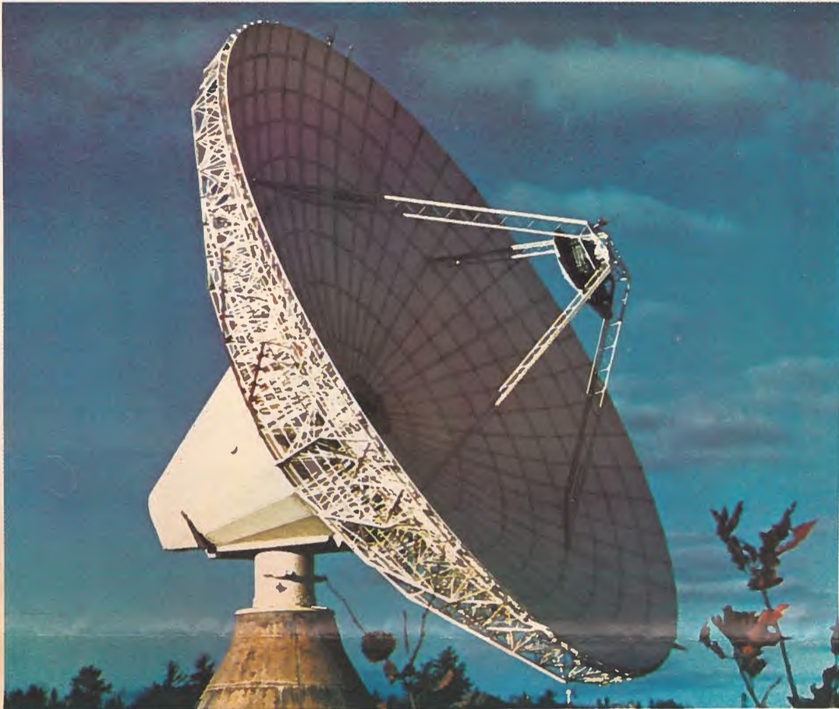
Antenna at Nova Scotia's Mill Village site for Canadian Overseas Telecommunications Corporation measures 97 feet (30 m) in diameter. This RCA earth station is used for satellite communications links and is one of several major earth station systems supplied to countries throughout the world by RCA.
