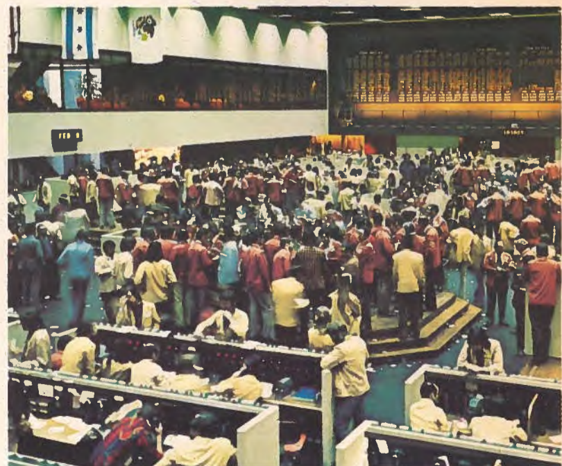
The Chicago Mercantile Exchange, the world's largest perishable commodity exchange, was installed in 1972 by the Electronics Division of Ferranti-Packard Limited, Toronto, Ontario. The complete system with two display boards each 74.5 feet long by 11 feet wide (22.7m by 3.4m) has 5,080 4.1-inch (104.1mm) high characters. Another exchange system recently installed by Ferranti-Packard is at the Sao Paulo Stock Exchange, Brazil.
