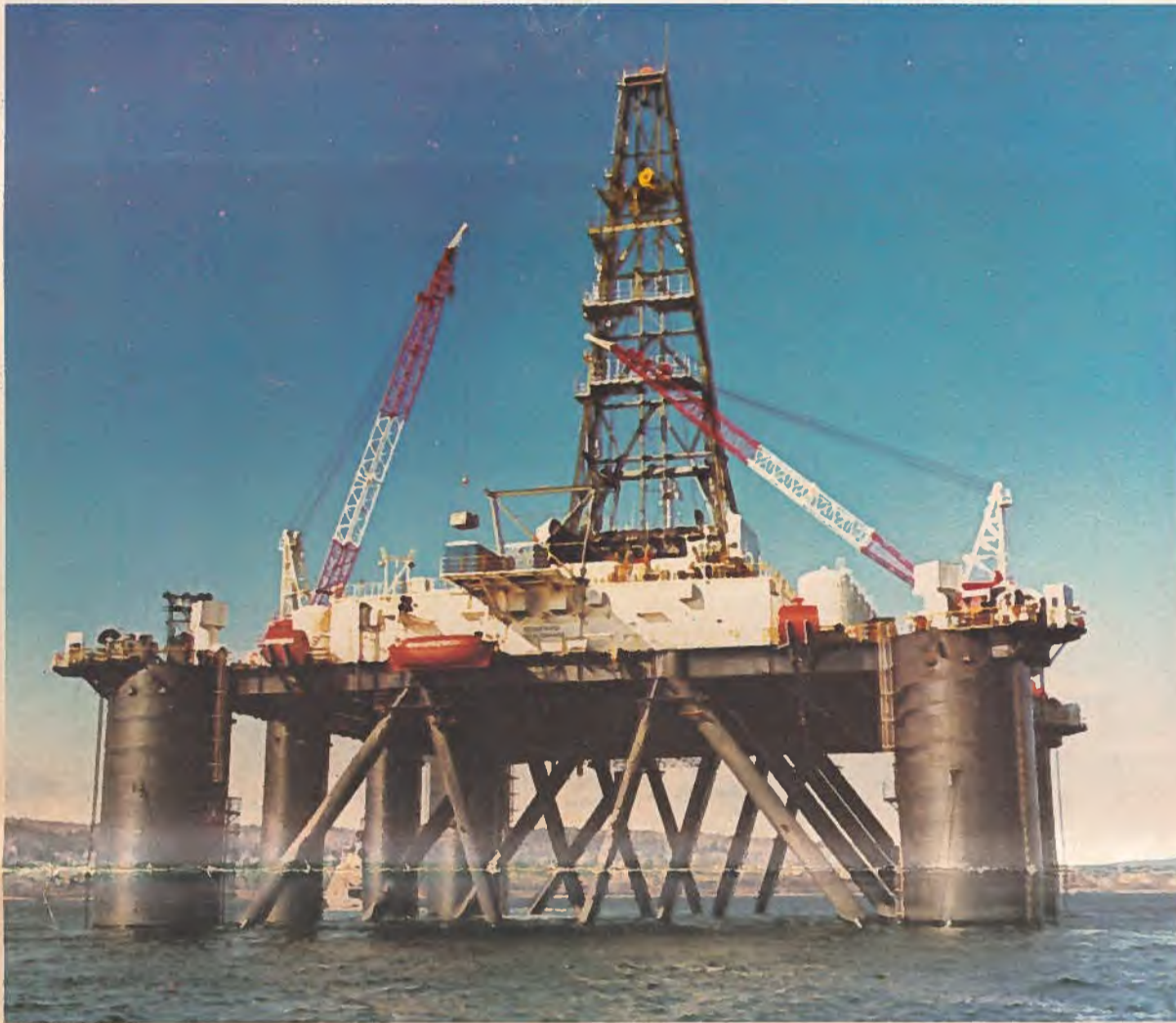
The Sedneth 701 is the fourth semi-submersible offshore drilling vessel constructed by Halifax Shipyards, a division of Hawker Siddeley Canada Limited. The Sedneth has successfully undergone sea trials and is assigned to search for petroleum in the North Sea. Halifax Shipyards is also noted internationally for its Sedco series of floating oil rigs — the largest of their kind in the world. The Sedco rigs, of triangular configuration, are capable of drilling in the floating position in depths up to 600 feet (182.8m) and are designed to withstand the most severe maritime conditions.
