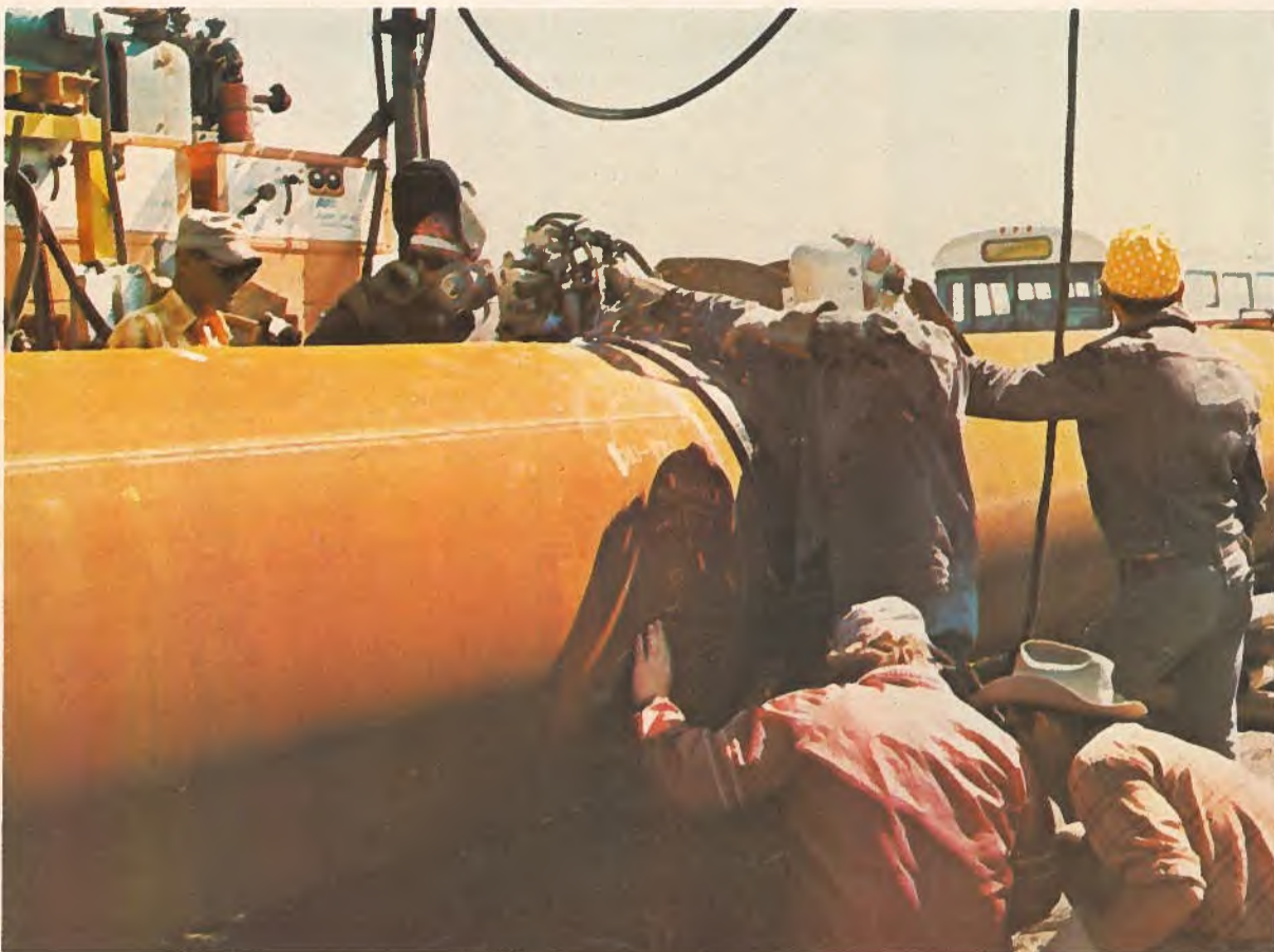
Employees of Alberta Gas Trunk Line Company are shown automatically welding 42-inch (106-cm) pipe.
