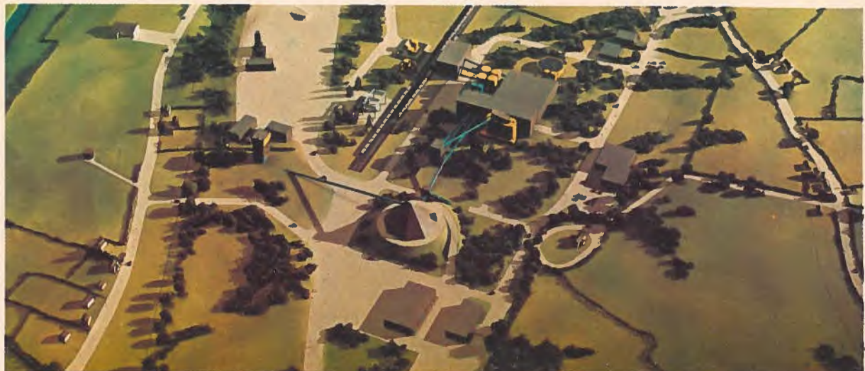
Model of the 7,500 tons per day zinc-lead concentrator of Tara Mines Limited in Navan, Ireland, for which Kilborn currently is doing the design, procurement and construction management.
