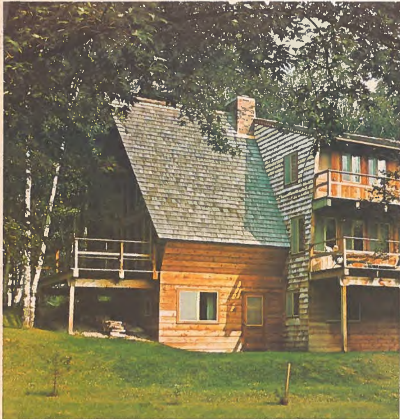
The most popular Nor-Wes chalet design, The Town and Country , has 1,140 square feet (105.9m 2 ) on the main floor and 660 square feet (61.3m 2 ) on the upper floor. Constructed of red western cedar from the forests of British Columbia, the model shown is located in Minneapolis, Minnesota. Highly adaptable, it features a cathedral ceiling.
