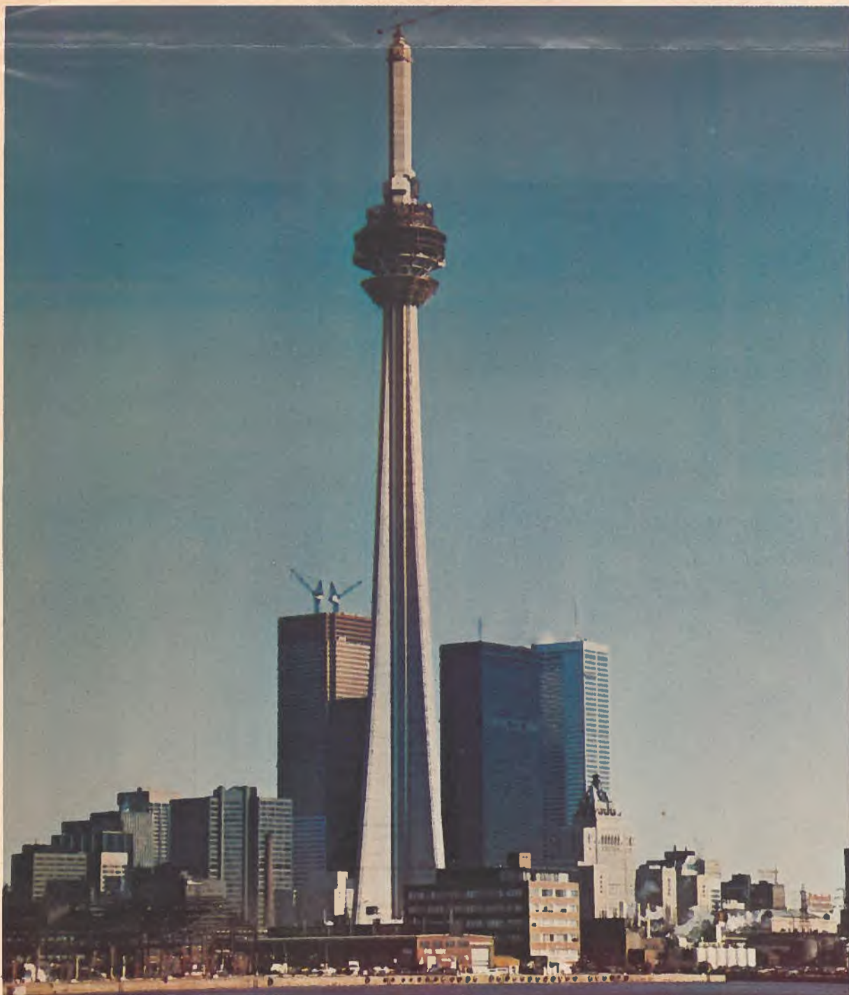
The C.N. Tower in Toronto, Ontario, is the world's tallest free-standing structure with a total height of 1,815 feet (553.2m). The 1,200 tons (1,088.6 metric tons) of steel that went into the 335-foot (102.1-m) high mast atop the tower were fabricated and erected by the Eastern Structural Division of Canron Limited, one of the Canadian companies participating in the Baghdad International Trade Fair in October 1975.
