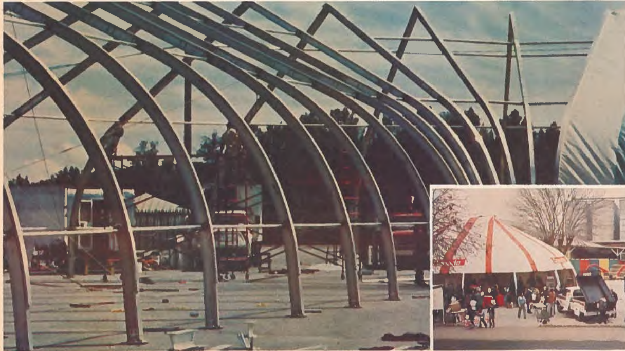
Erection and dismantling of Sprung structures is simplicity itself, with the use of lightweight beams and stressed membrane fabric. Since they are also compact for easy shipping, Sprung Instant structures are being widely used to house the products of Canadian exhibitors at international trade shows. Used this past spring at the California Farm Show (inset), Sprung structures will also house Canada's exhibits at the Algiers International Trade Fair and the Baghdad International Trade Fair. Code 3-165
