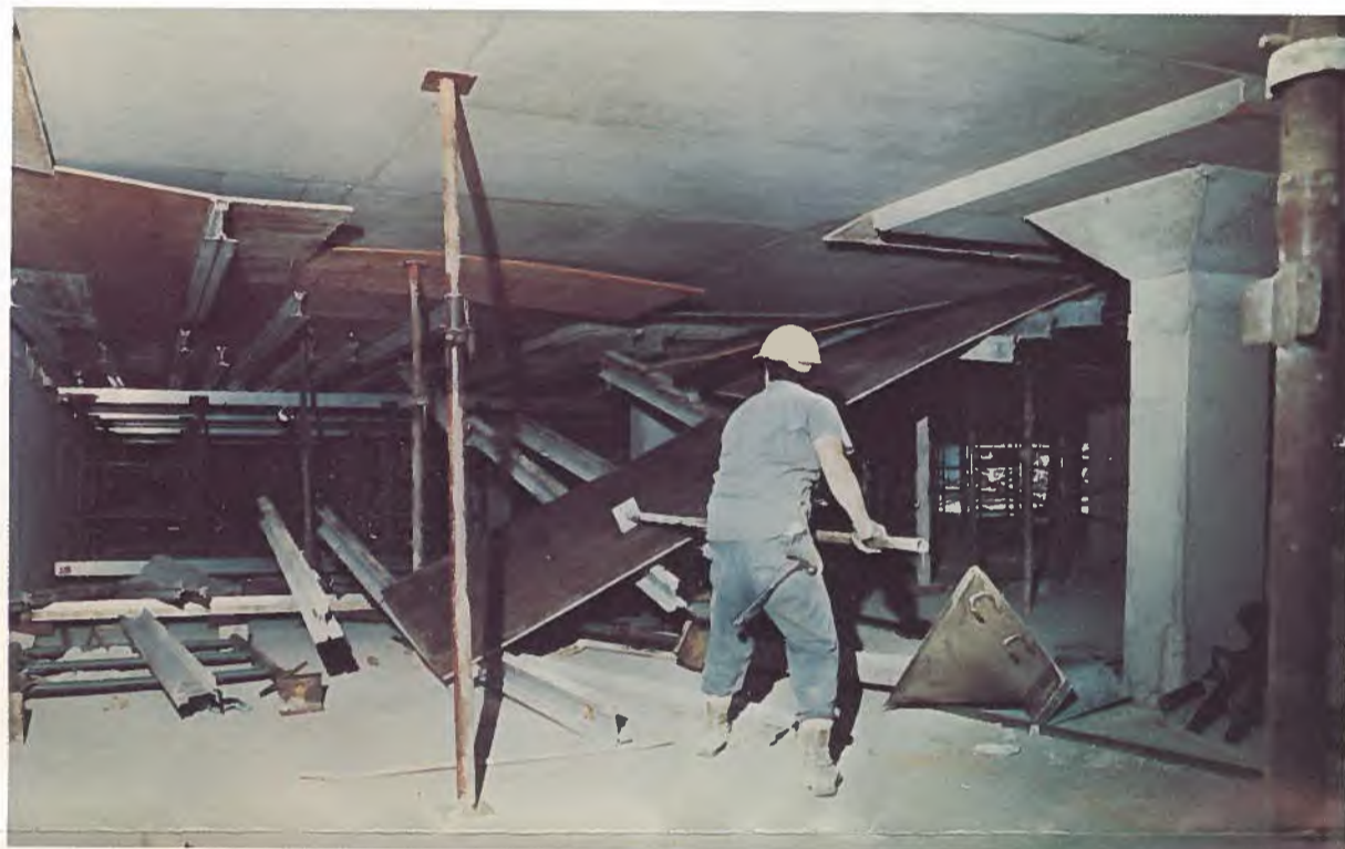
Dismantling Aluma's stationary forming system is fast and easy. When the concrete has reached the required strength, the single-shore poles that temporarily support the underfloor forms are simply knocked or pulled away. The whole sub-floor assembly then drops to the ground, where it can easily be sorted out and picked up by workmen.
