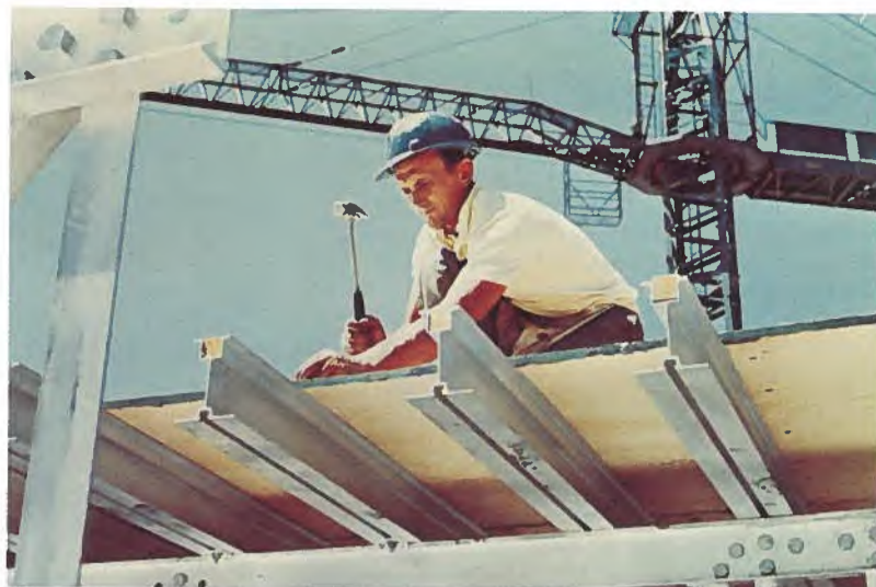
Concentrating on the job at hand, this workman secures the flooring to the nailing strip on the aluminum stringers as the final step before concrete is poured.
