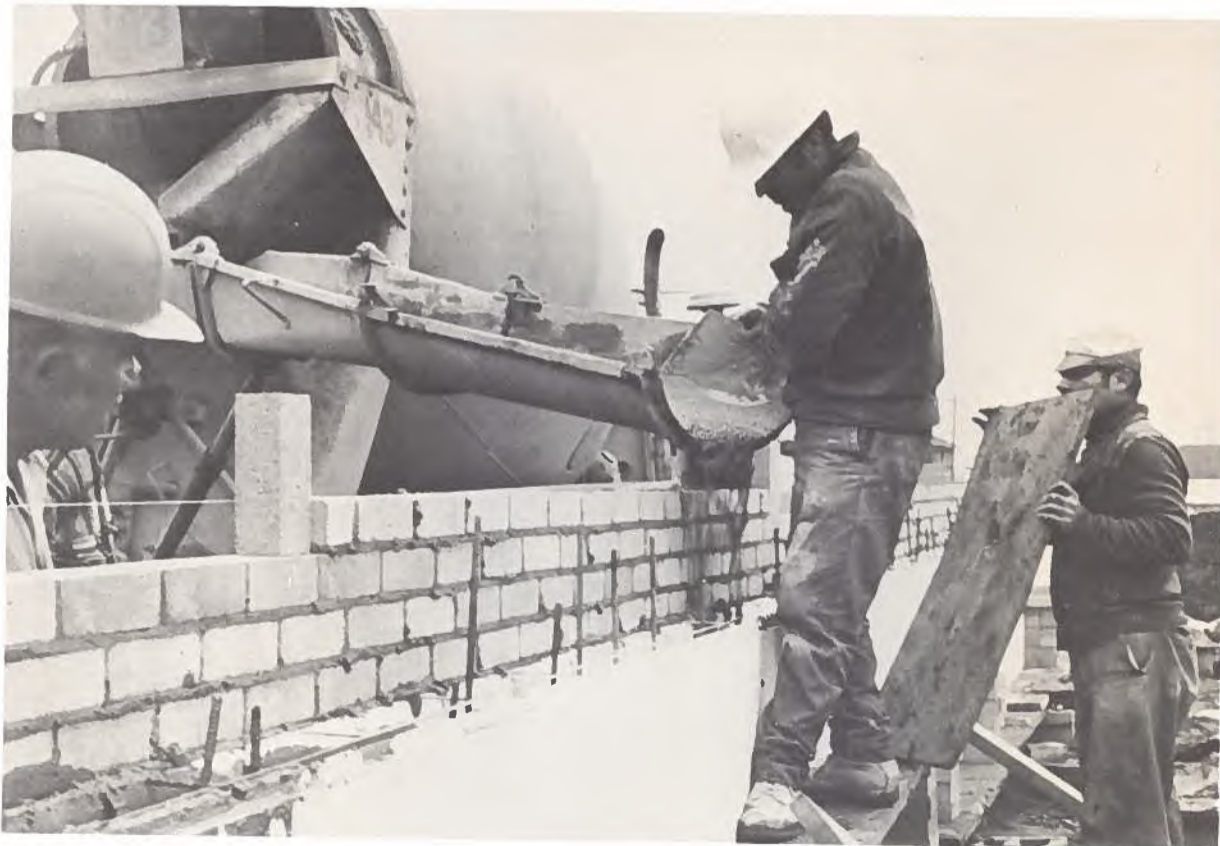
These men are busy pouring concrete into Foam-Form, a hollow core, polystyrene block made by a subsidiary company of Universal Sections, Foam-Form Canada Ltd. The blocks, which are stacked in courses like brickwork to make a wall, act as a form to receive poured concrete. After the concrete has cured, they remain in place to provide high quality insulation over a continuous reinforced concrete wall.
