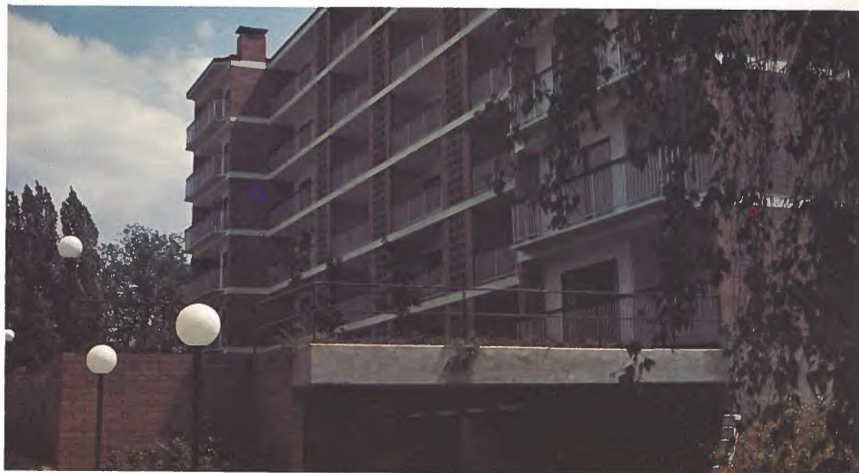
The finished product — an attractive lowrise building that used Dy-Core slabs for economical value.
