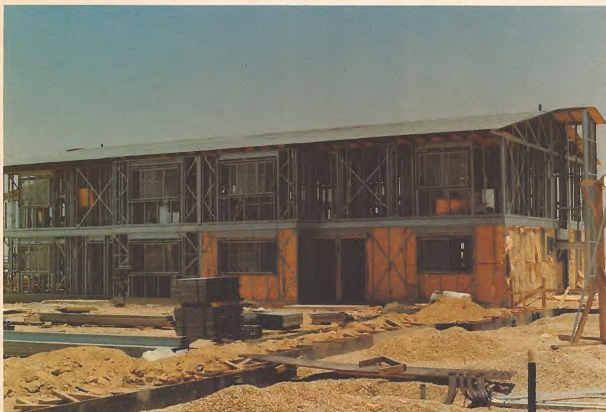
Using the Domfab Thermobuilt System of construction, Domfab Ltd. of Montreal, Quebec, supplies a wide range of custom-designed buildings — up to five storeys high — to international clients. The simple and easy-to-erect system uses steel wall structures that are separated by exterior and interior skins that are fire resistant, improve insulation and prevent humidity and condensation. Domfab Ltd. is extremely active in Saudi Arabia where it is working on several major projects including King Khaled Military City and the Jubail Industrial Complex.
