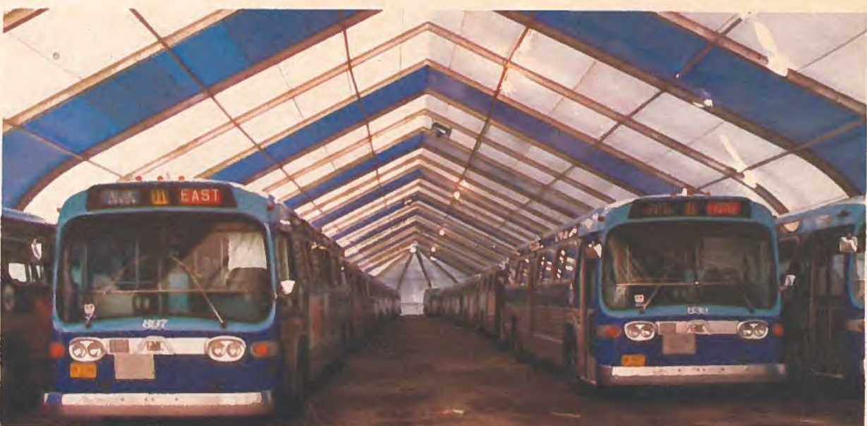
Sprung Instant Structures has established its proven worth in virtually every segment of industry. From elegant exhibitions and automotive showrooms to rugged workshops and warehouses — Sprung has covered them all. Here the 18 m x 107 m (60 ft. x 350 ft.) structure is used as a bus depot.
