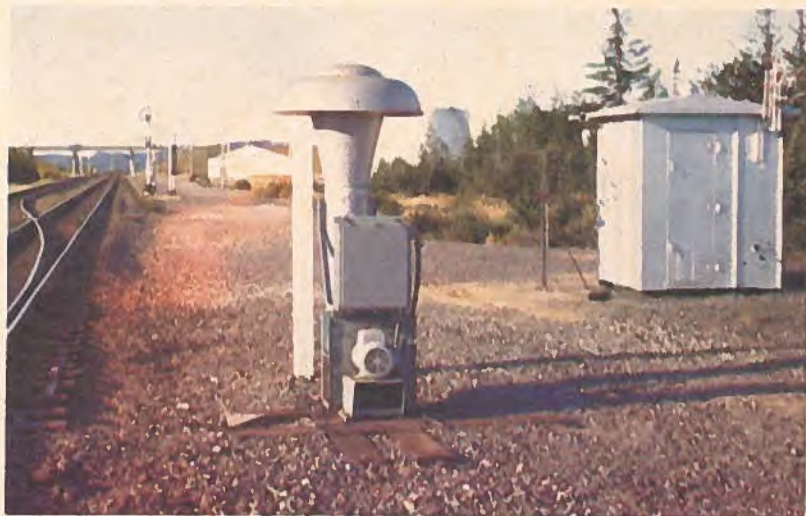
The horizontal air curtain \Delta and the hot box detector protector system are just two of the units manufactured by Hovey & Associates (1979) Ltd. of Ottawa, Ontario, for cost-effective use by the rail transportation industry.
