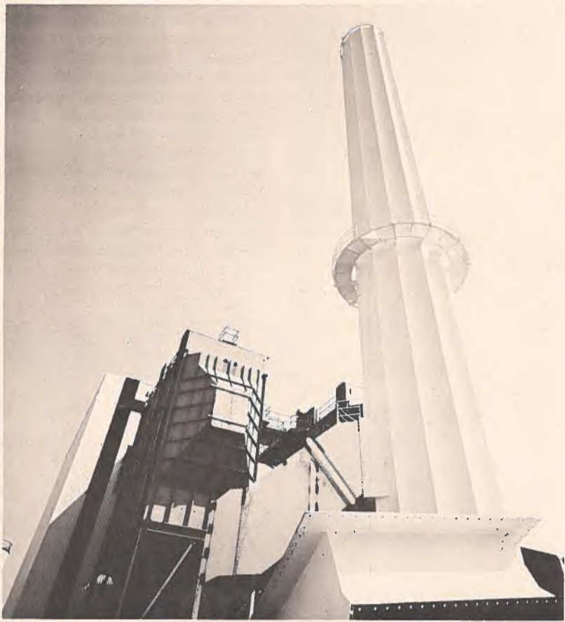
This isn't really a Grecian column but a dual-flue, hermetically sealed smokestack for the boilers of Sutin's new steam-producing garbage disposal system.
