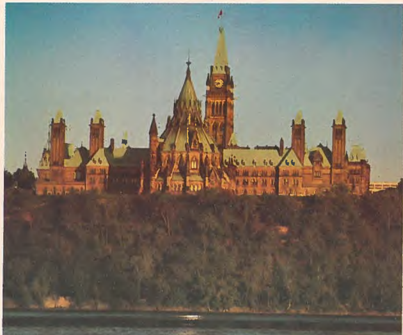
Canada's Parliament Buildings in Ottawa at sunset, with the Ottawa River in the foreground.
