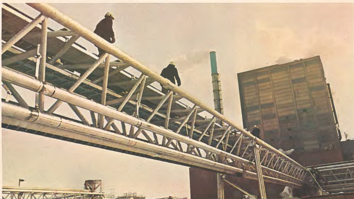
Strong, lightweight aluminum-pipe bridge erected by Dominion Aluminum for a Nova Scotia pulpmill.
