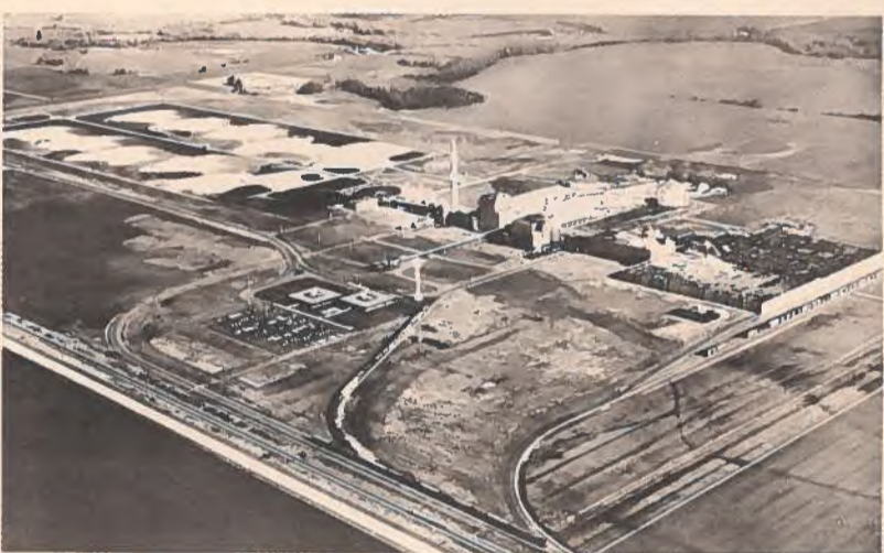
Sandwell developed the design, designed detail and supervised construction of this American Can Company 300-ton-a-day bleached-kraft, pulp, paper and tissue mill in Halsey, Oregon. Code 3-4
