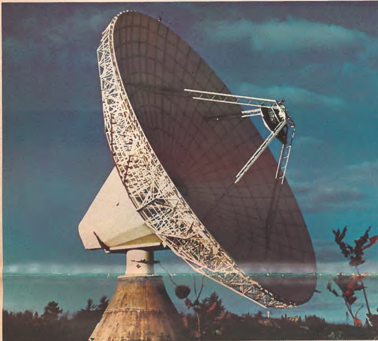
Antenna at Nova Scotia's Mill Village site for Canadian Overseas Telecommunications Corporation measures 97 feet (30 m) in diameter. This RCA earth station is used for satellite communications links and is one of several major earth station systems supplied to countries throughout the world by RCA Limited, Montreal.
