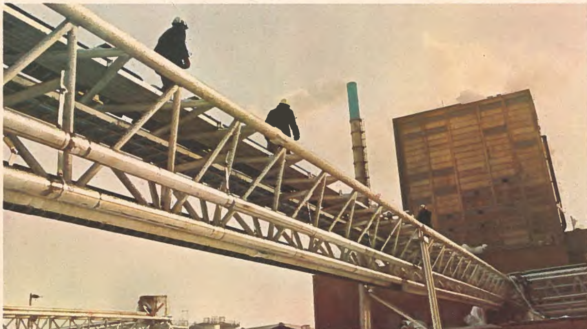
Strong, lightweight aluminum-pipe bridge erected by Dominion Aluminum for a Nova Scotia pulpmill.
