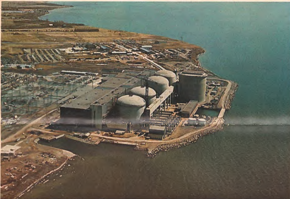
Two of the four units of Pickering nuclear-power station are already supplying more than 1,000,000kw to Ontario Hydro system.
