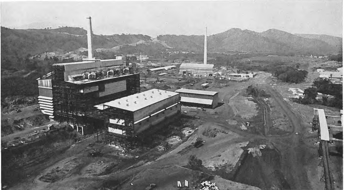
Falconbridge is investing nearly $200 million in the Dominican Republic to mine and process extensive ferro-laterite ore deposits. Its plant, near the town of Bonao, is nearing completion and should soon be in full production.
