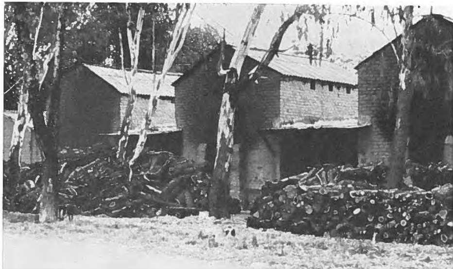
Clay adobe drying kilns in the Province of Salta in Argentina. These are wood-burning kilns with metal roofs and are not insulated. Other structures would have to be built if Canadian drying equipment is to be used there.
