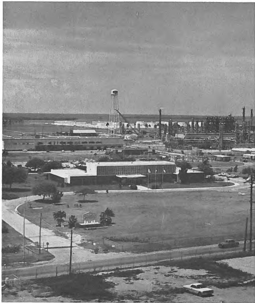
Sprawled over a large acreage, the Union Carbide plant is representative of the many giant complexes that have been built by international firms on Puerto Rico's south coast. Over the years, the petrochemical industry has contributed most to the island's economic growth and now has an investment of $1 billion.
