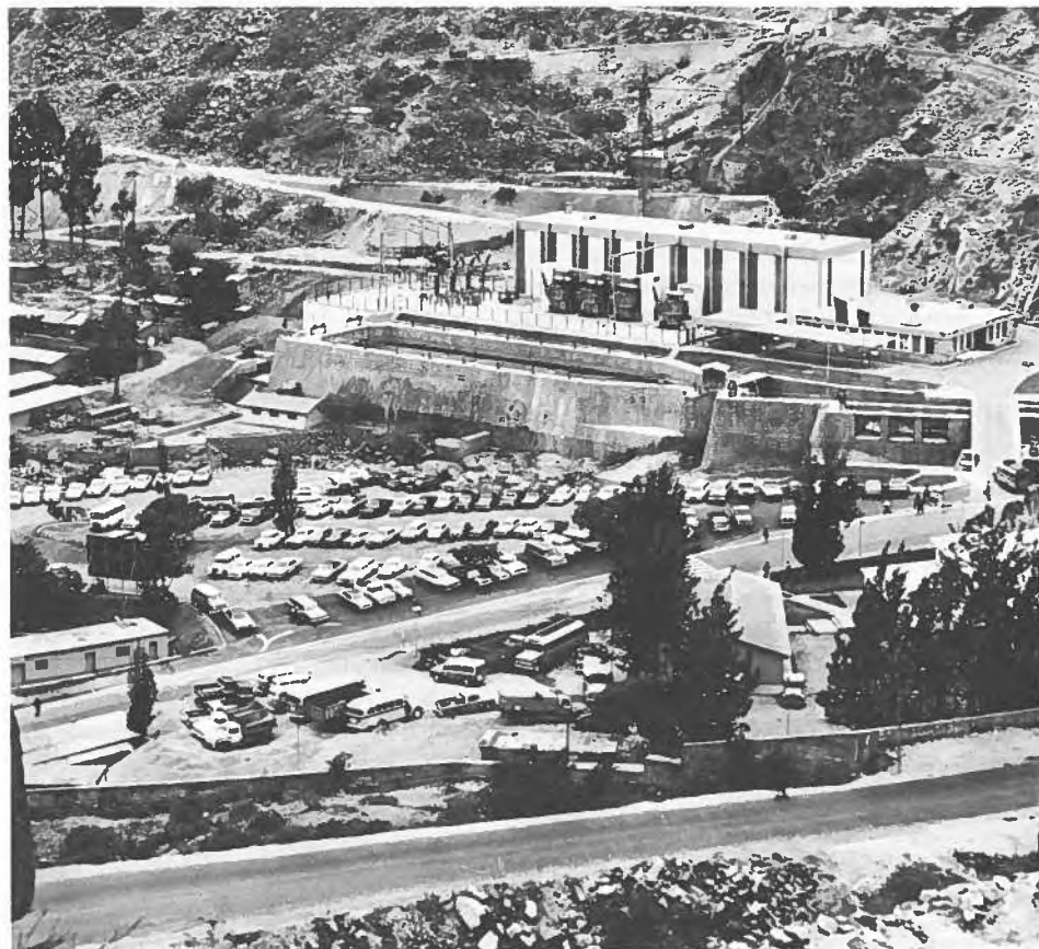
Looking down on the new Pablo Boner hydroelectric plant located high in the Andes about 60 miles east of Lima. The plant was brought on stream in 1971, thereby increasing the total capacity of Empresas Electricas Asociadas to more than 500,000 kw.
