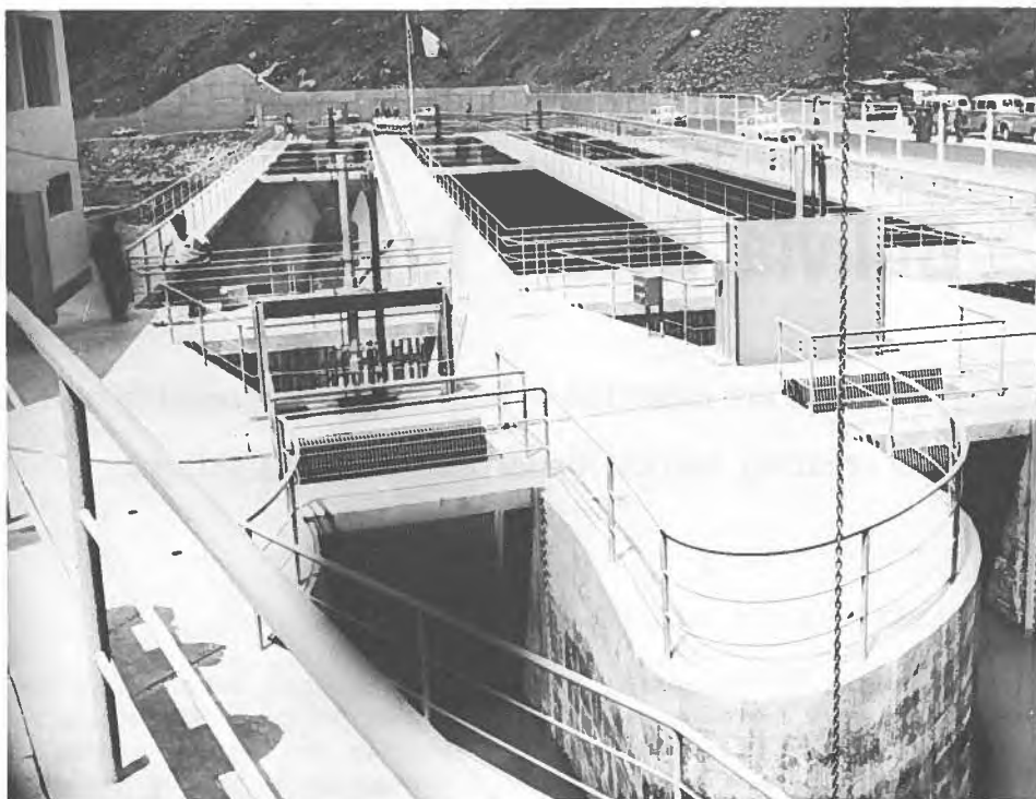
Raised intake gates (at right in photo) indicate water is flowing through two of the artificial passages in the forebay of the Pablo Boner hydroelectric plant near Lima. The plant is named after the man who planned and directed the expansion of Lima Light and Power Company (now Electricas Asociadas) during the past 40 years.
