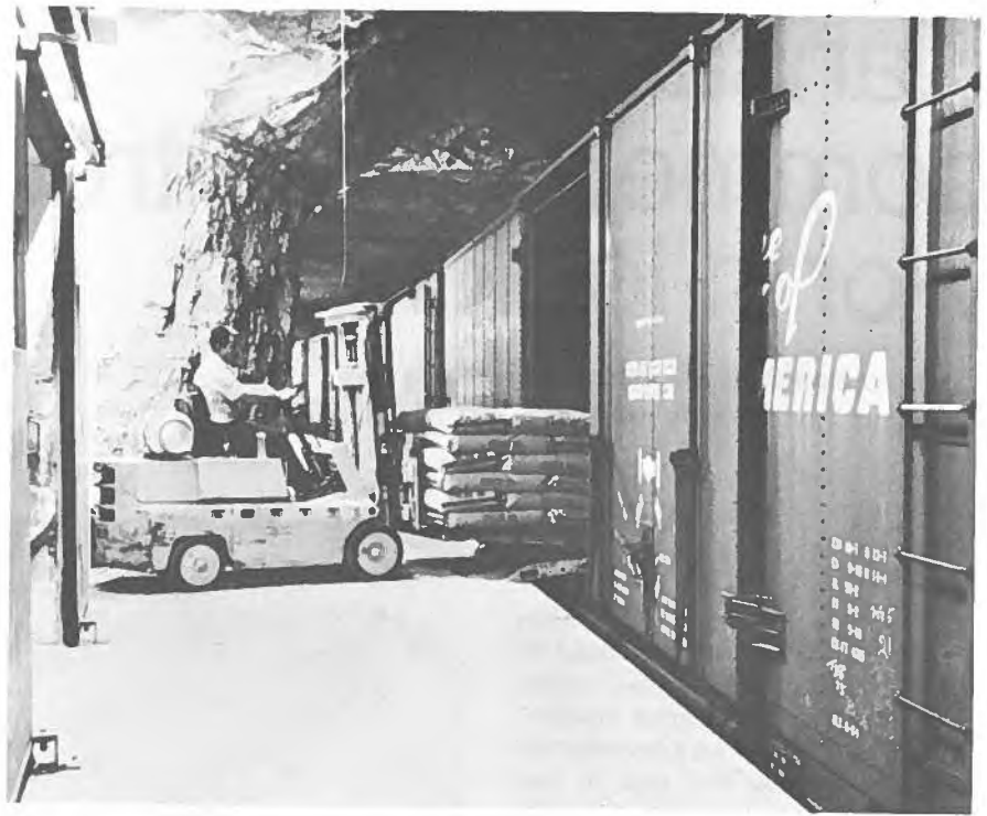
Excavated from limestone deposits, these caverns provide cheap, clean storage facilities just seven miles from downtown Kansas City. Both road and rail transport can unload their cargoes right at the storage area.
