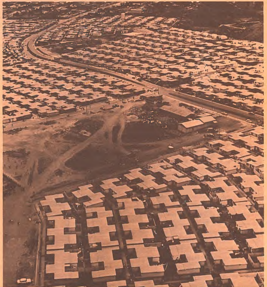
Low-income housing units are relieving housing shortages for Central America's burgeoning population. This 5,260-unit development in Guatemala was partially financed by a $5.3 million Inter-American Development Bank loan and is available to families earning $40 to $140 monthly.
