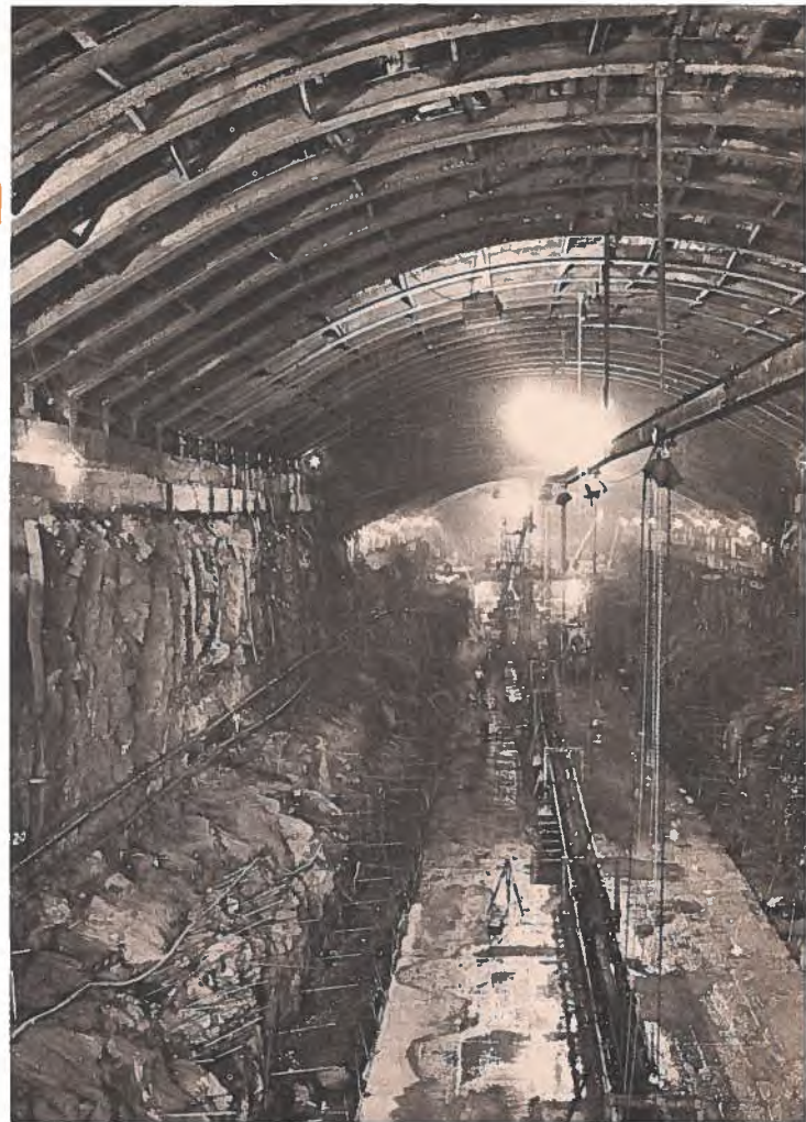
This tunnel being built under the East River is part of the New York City subway extension program. Steel being used in the tunnel is provided by a Canadian firm.
