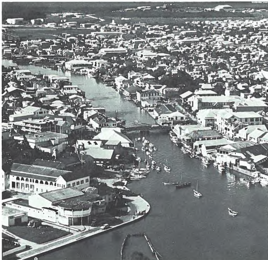
Part of Belize City. Another medium-size hotel may be built here in the near future.
