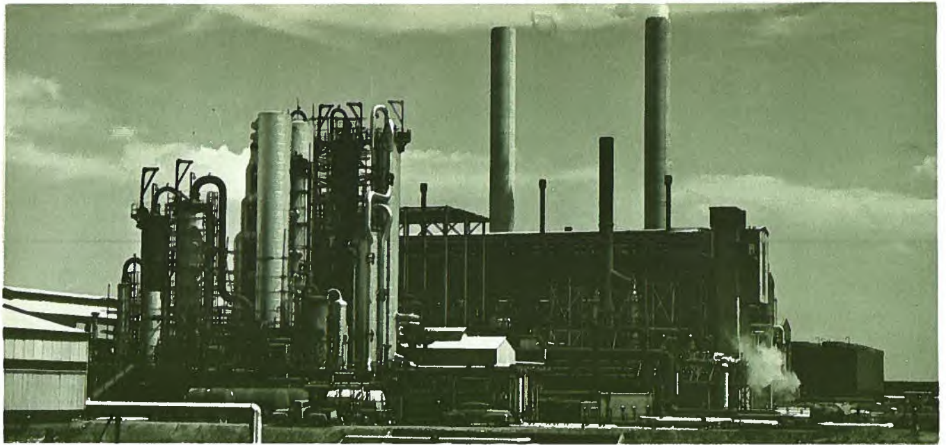
SASOL — the world's largest oil-from-coal plant.
