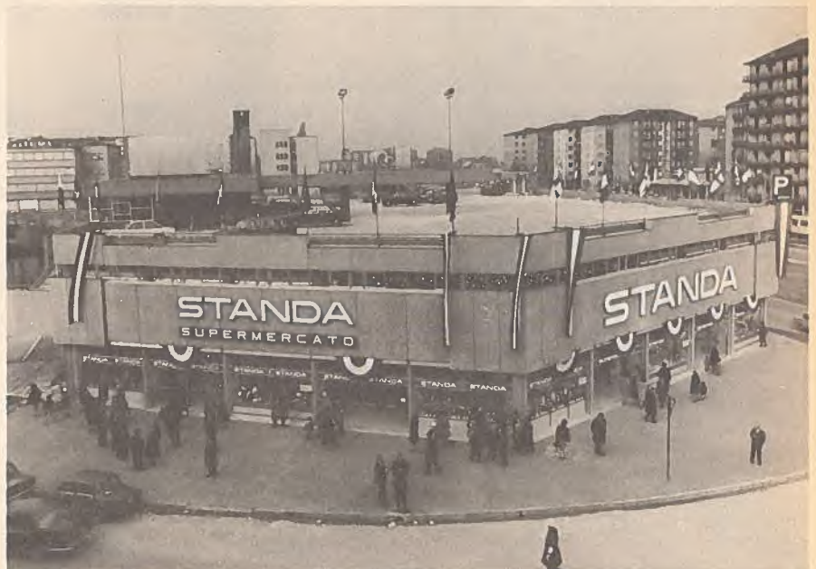
One of the new Standa stores in a Milan suburb. Note rooftop parking.
