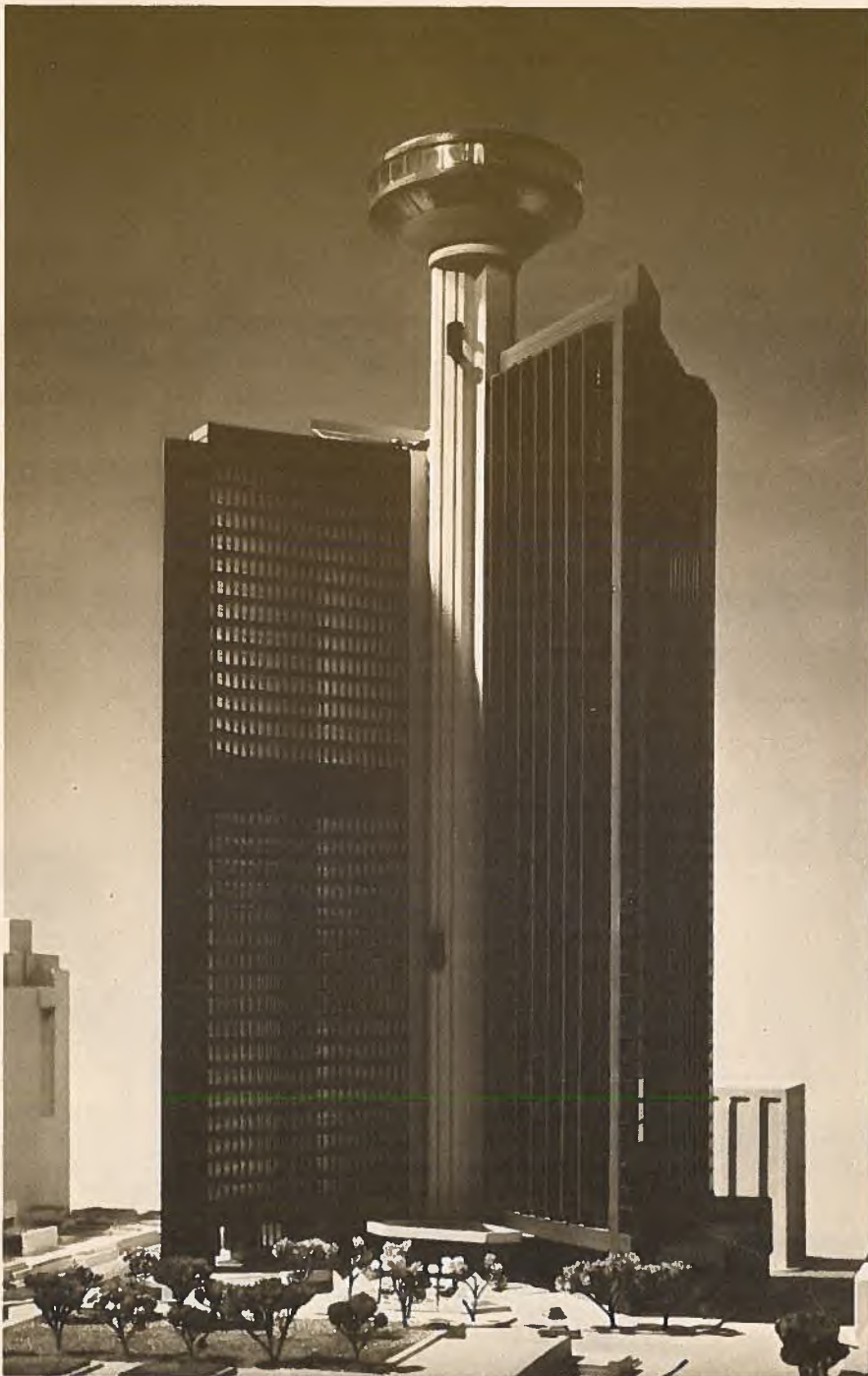
The 48-storey hotel to be built in Montreal by Concordia Estates Ltd. will have two panoramic elevators running on the outside of the central tower.
