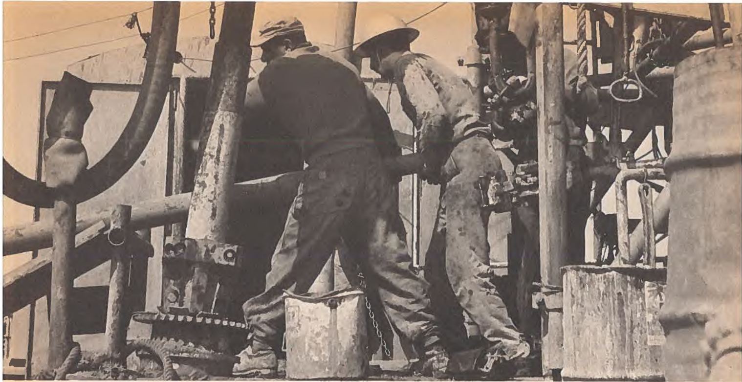
Drilling operations in the desert, this time for water.
