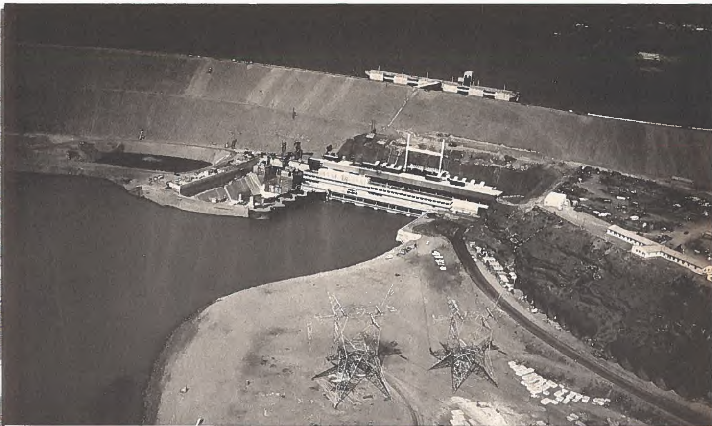
Part of the dam and tailrace at the El Chocon site.
