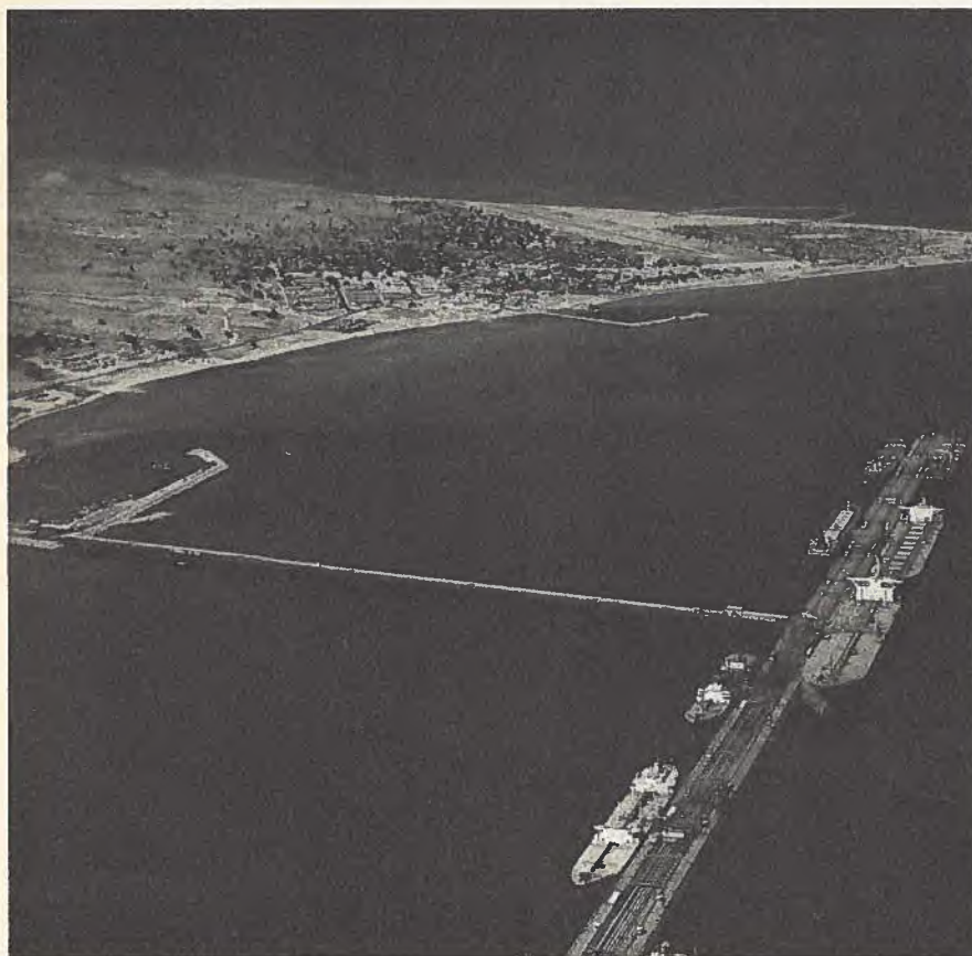
The 10-berth, T-head jetty of the Kharg Crude Oil Export Terminal.
