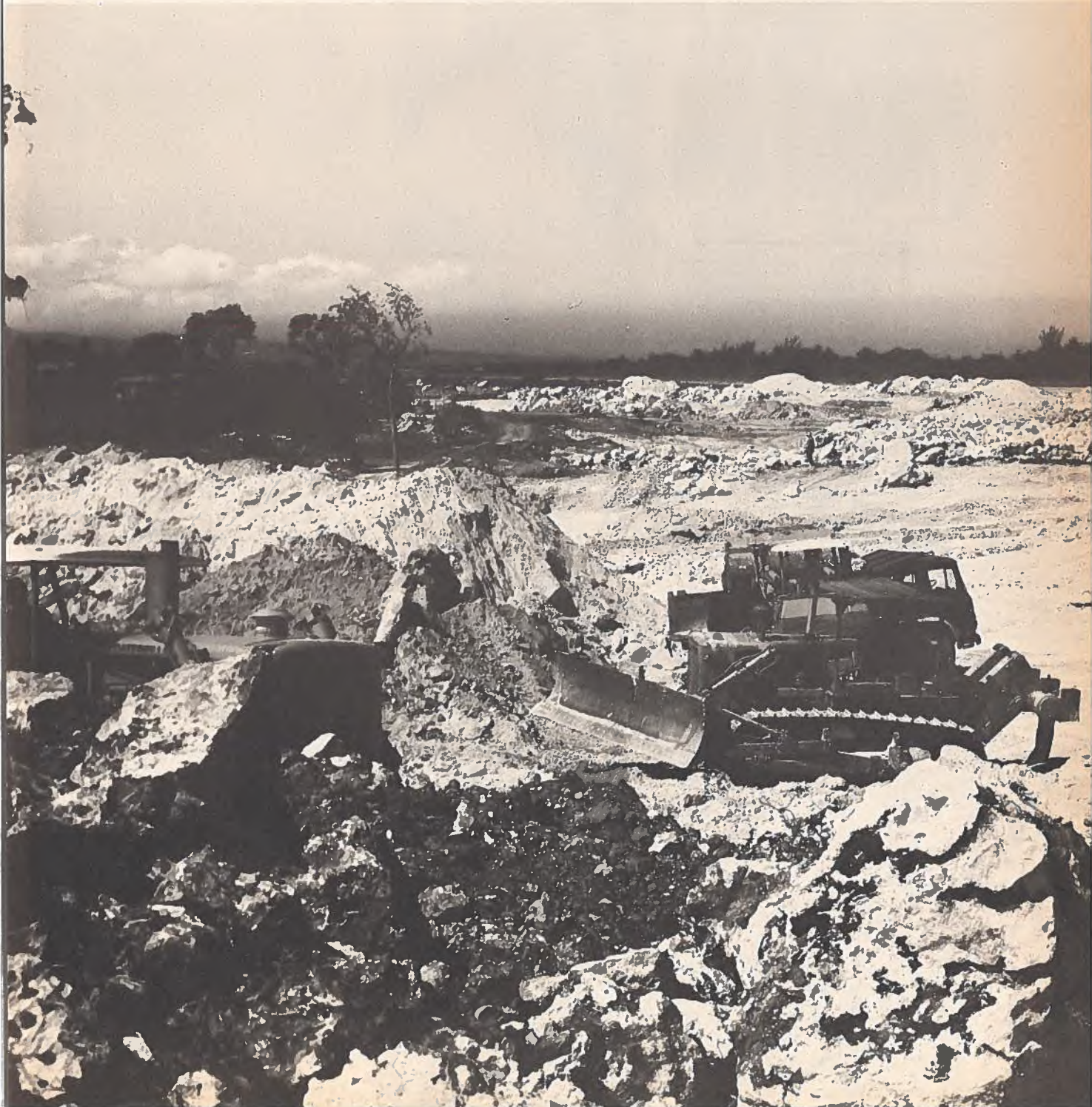
Highway construction between Kingston and Spanish Town.
