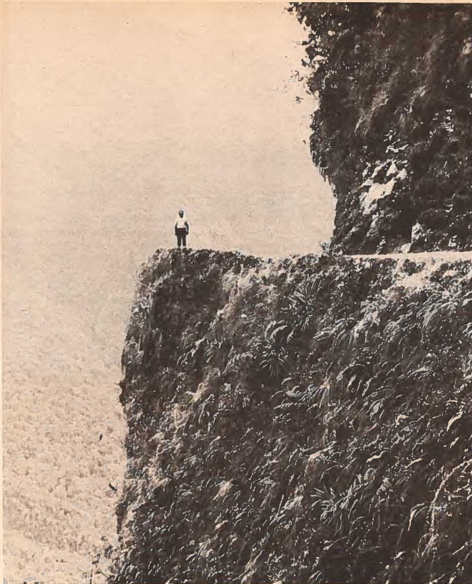
Highway project, Bolivia
