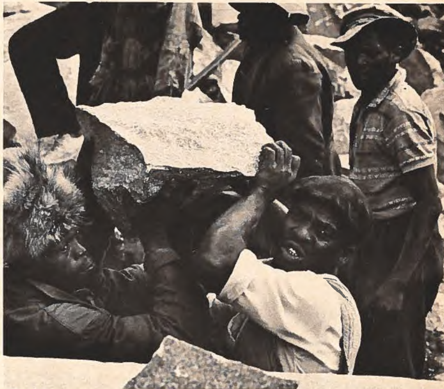
Swazi workmen load rock on to a truck during roadwork.
