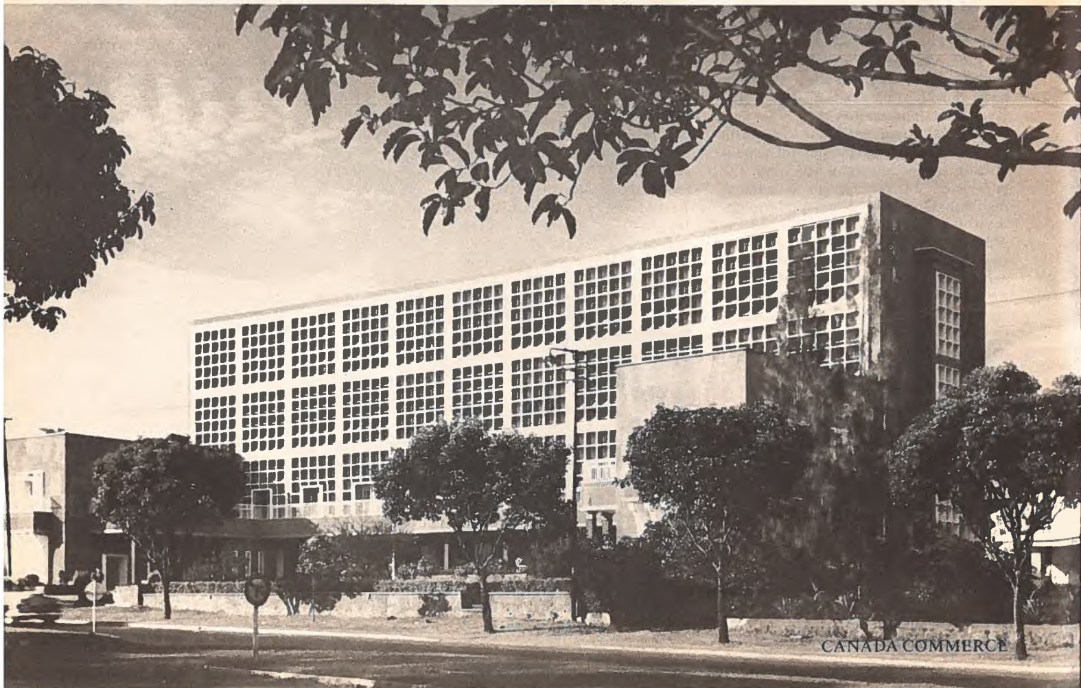
Modern buildings and tree-lined streets greet the visitor to Djakarta. This is the Central Office for Agriculture
