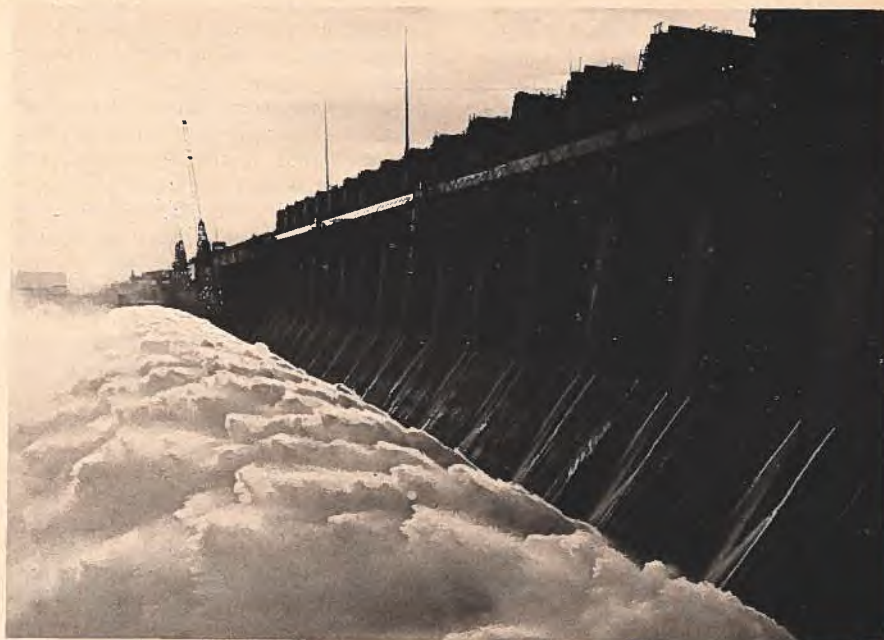
The Ilha Solteira will eventually have 20 turbines and, together with another station just downstream, will make the Urubupenga complex capable of producing 4.6 million kw.
