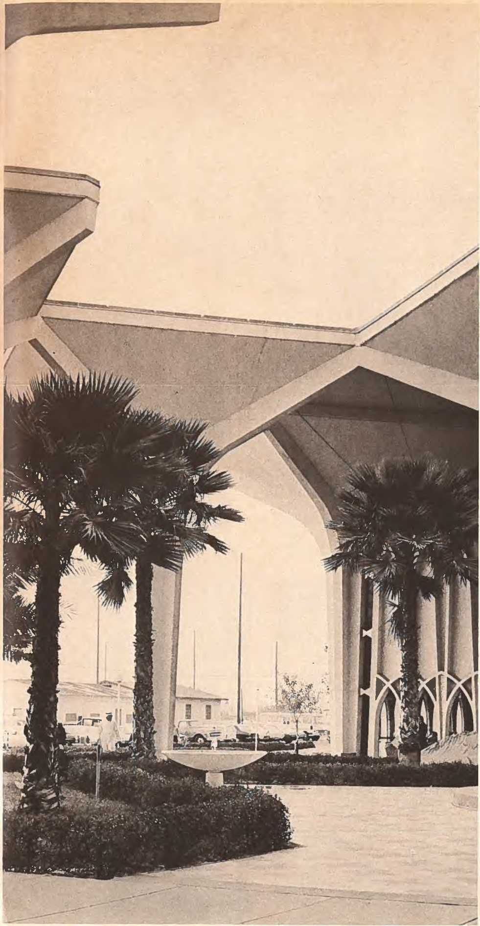
Part of the main building of the Dhahran o airport.
