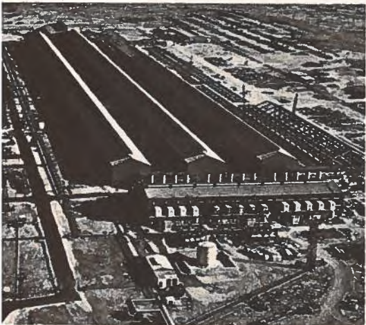
Bahrain's industrial expansion includes this aluminum smelter, which is the largest in the Arab world.
