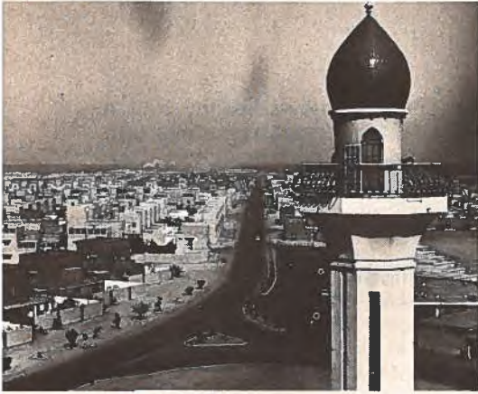
Issa Town, Bahrain — part of a housing program to accommodate 35,000 people.
