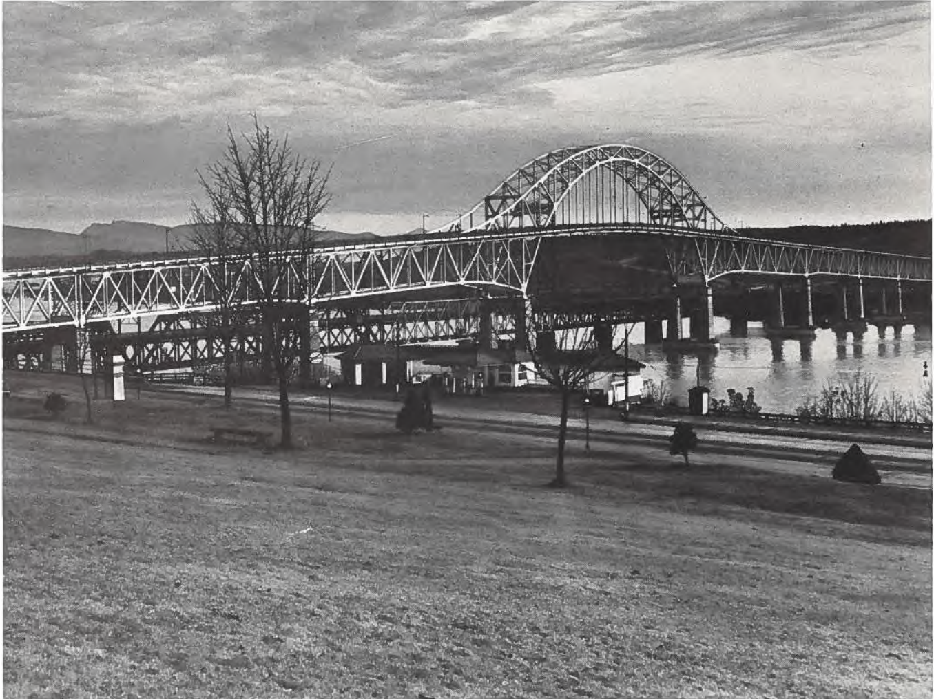
Patullo Bridge, British Columbia — one of Swan Wooster's first projects.
