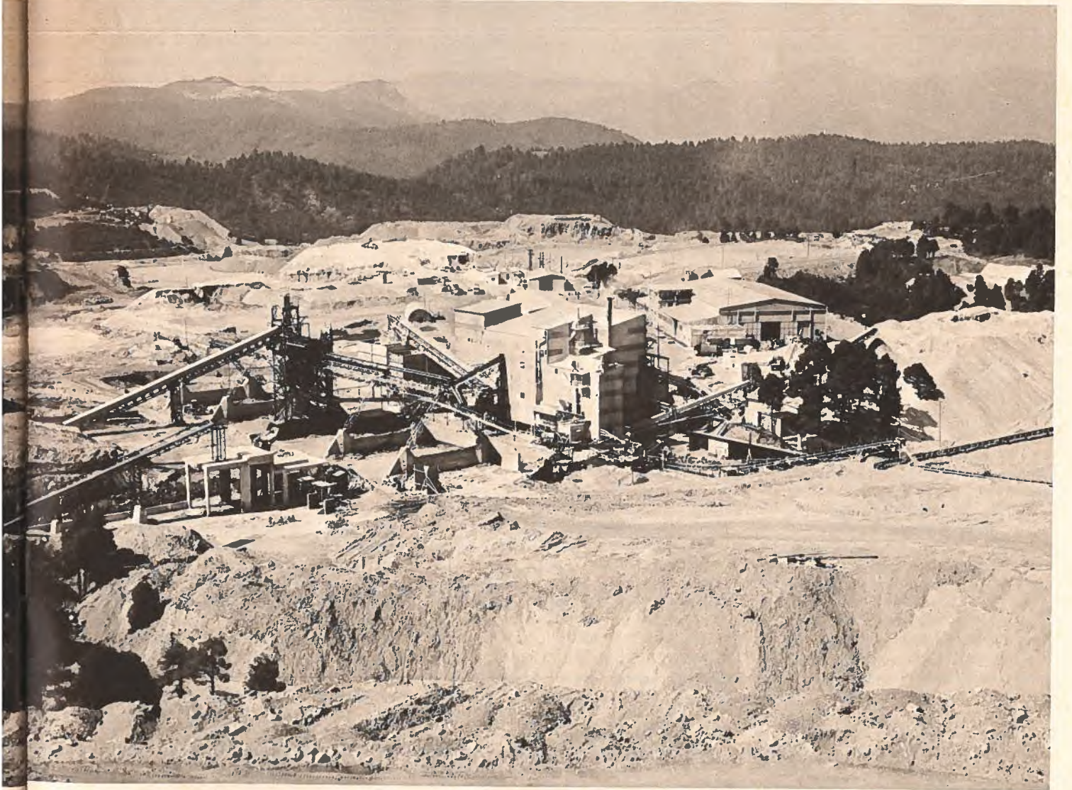
with a capacity of 1,000 metric tons an hour of deadburnt magnesite.
