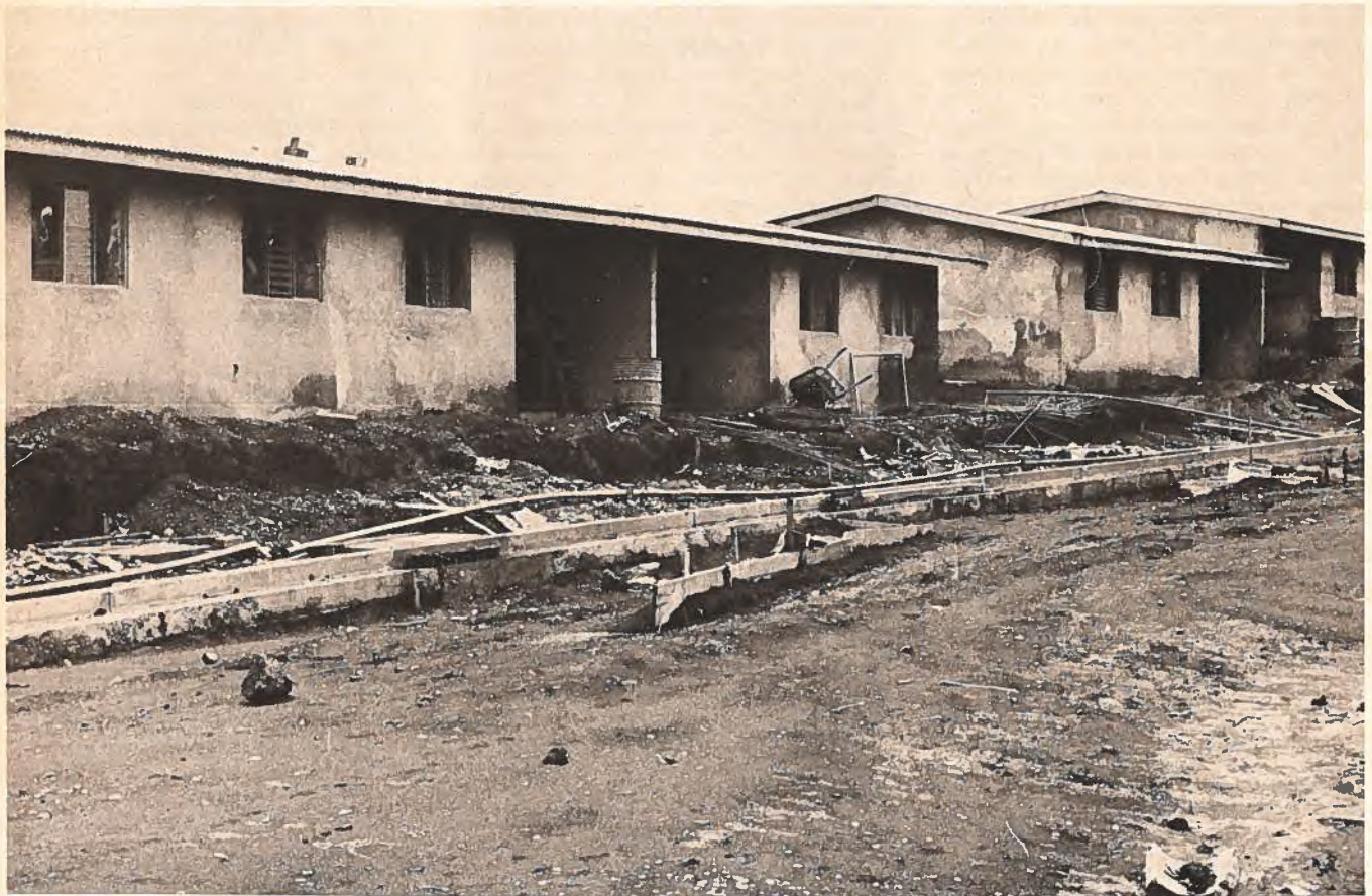
Low-cost housing under construction near San Jose.
