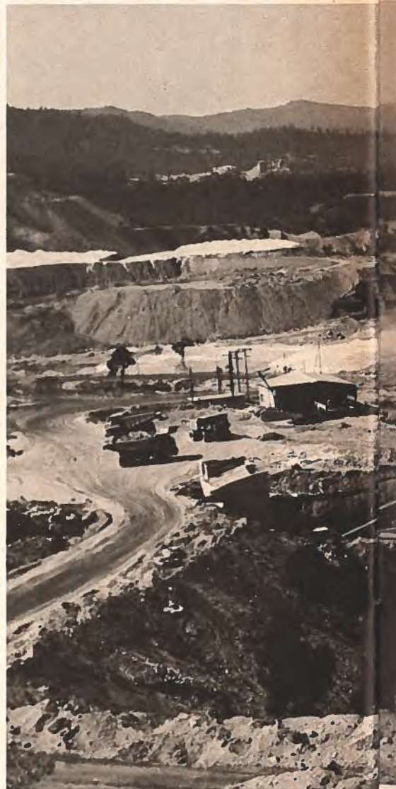
The magnesite dressing plant at Kakavos, Euboea.
