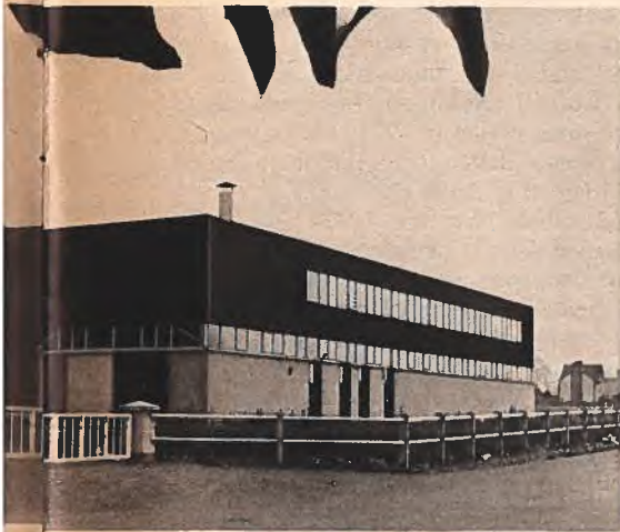
A ready-made factory built by the Irish Industrial Development Authority and typical of those offered to incoming industry.
