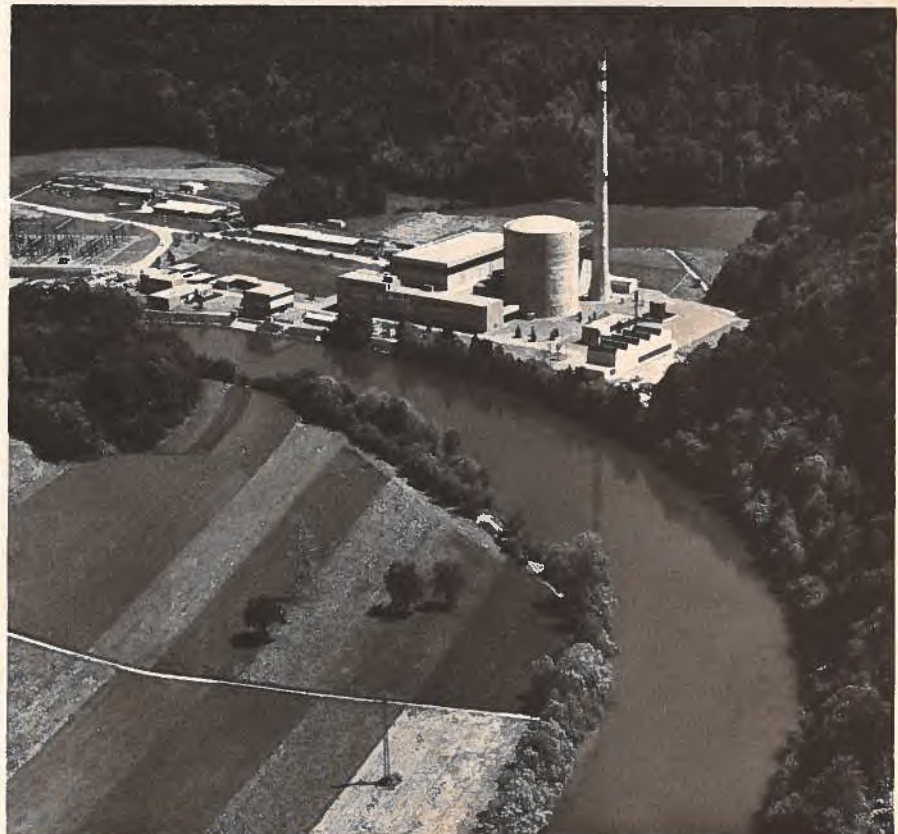
The 306-MW Muhleberg nuclear power plant near Berne, owned by Bernische Kraftwerke AG.
