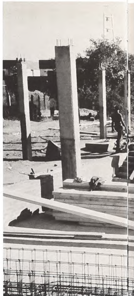
Botswana Museum under construction
