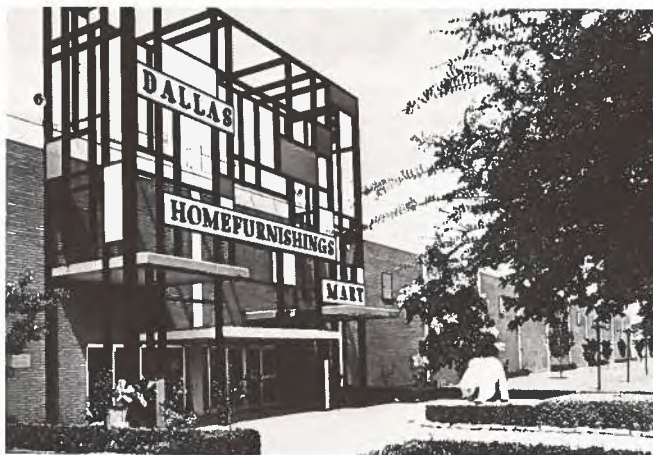
The Dallas Homefurnishings Mart was designed for the most advantageous display of furniture. Broad hallways, courtyards and winding stairways give visibility to showrooms on both floors while special lighting, acoustical ceilings and resilient flooring add to the gracious atmosphere.
