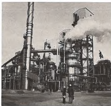
The new refining plant of Gulf Oil Canada Limited.
