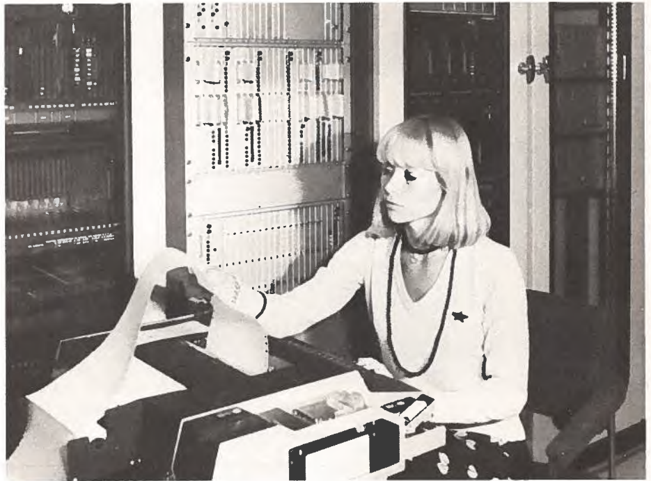
Switch of the Transpac data transmission network which uses the package communication technique.
