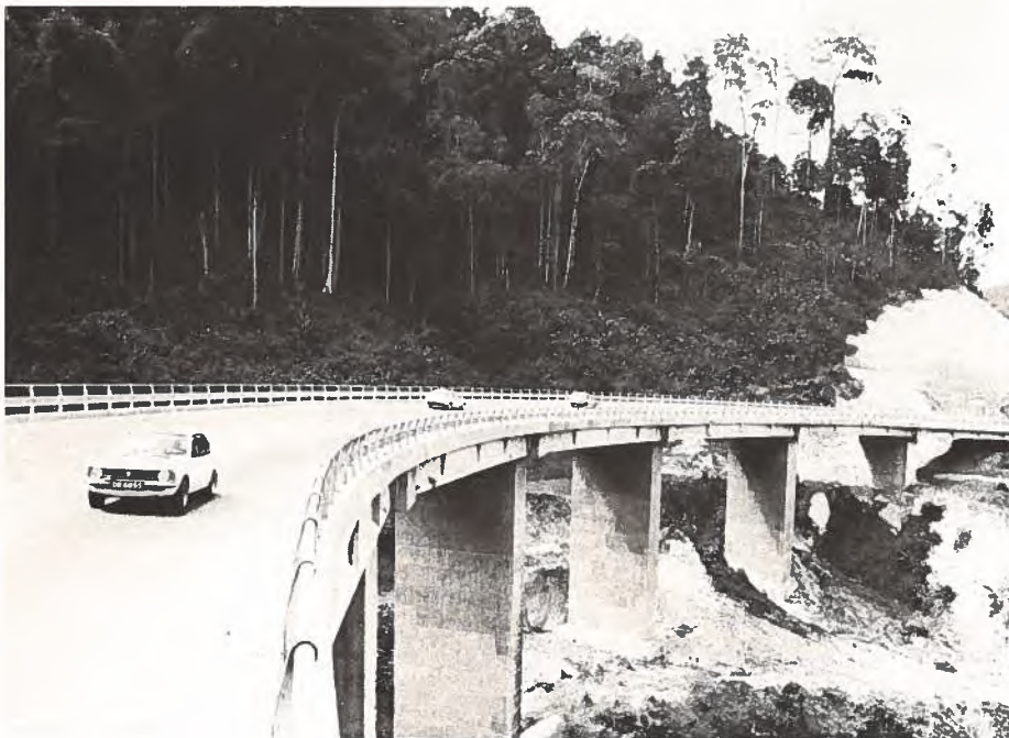
Constructed in the State of Selangor in the vicinity of Genting Sempiah, the 85 km Kuala Lumpur-Karak Highway leads through a 914 metre single-bore tunnel.
