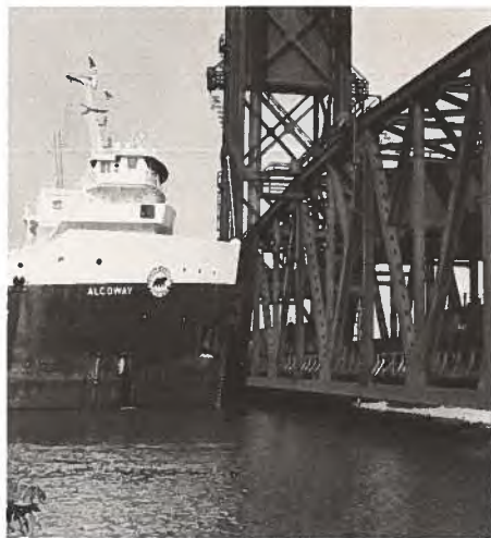
Canadian ore carrier waits for the famous Baltimore-Ohio rail bridge to open.
