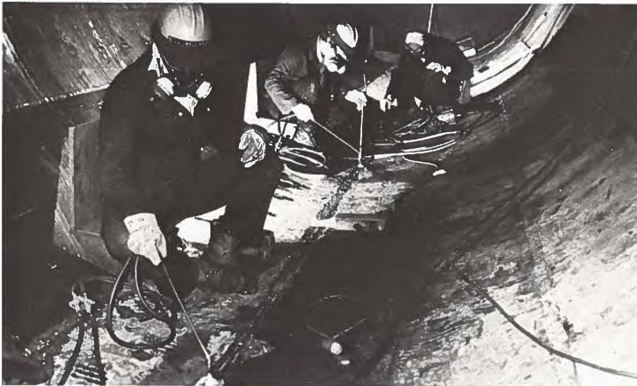
Cominco workers rush the completion of the zinc pressure leaching installation at Trail, top, completing the observation decks, and below, installing the lead lining in the autoclave (pressure vessel).
